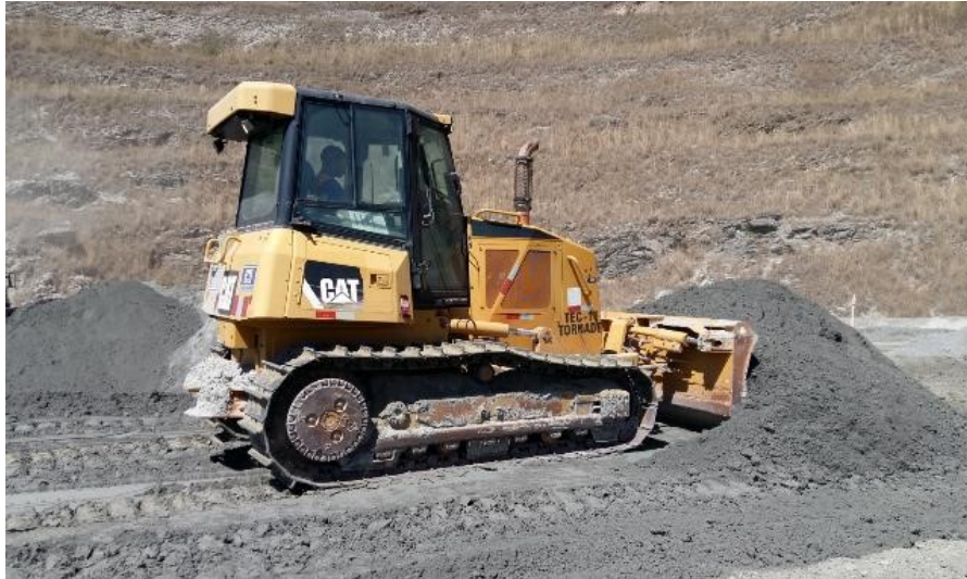
Figure 2 Spreading the material with a bulldozer (BVP Engenharia 2017)
