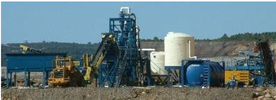
Figure 6 Mobile soil washing plant (ART Engineering 2018)
