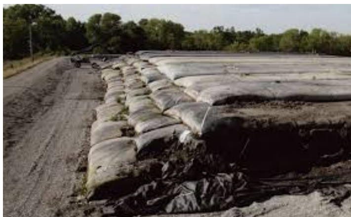
Figure 4 Geotube dewatered sludge (TenCate 2019)
