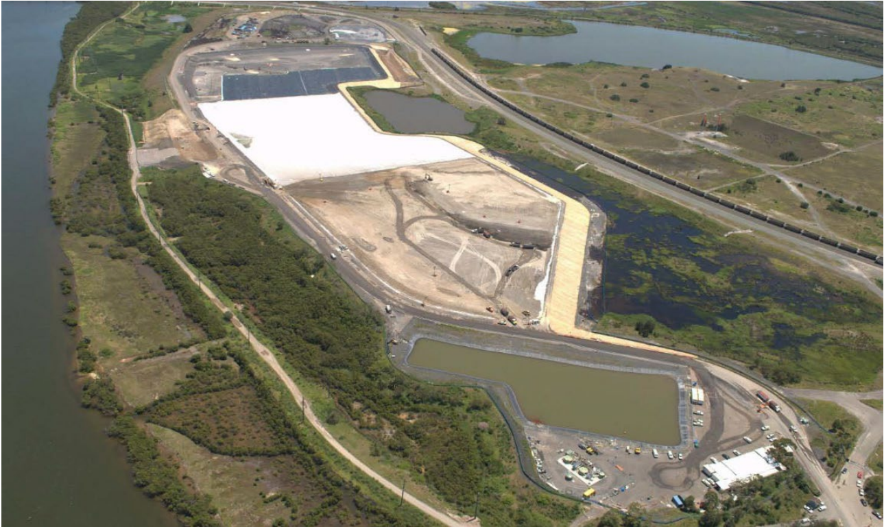
Figure 2 Construction (circa November 2010) of the emplacement facility at Kooragang Island
