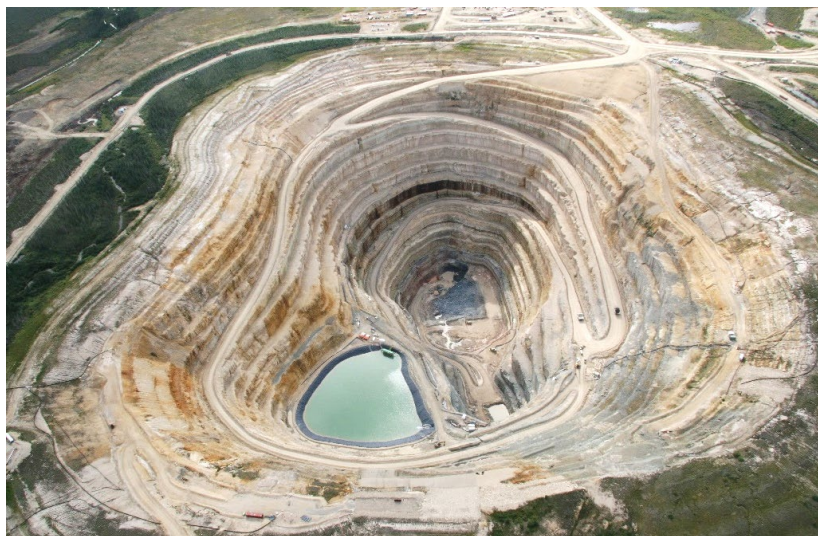
Figure 6 Photo showing overview of Victor Mine looking northeast. Note shallow overburden slopes and excellent limestone slope performance
