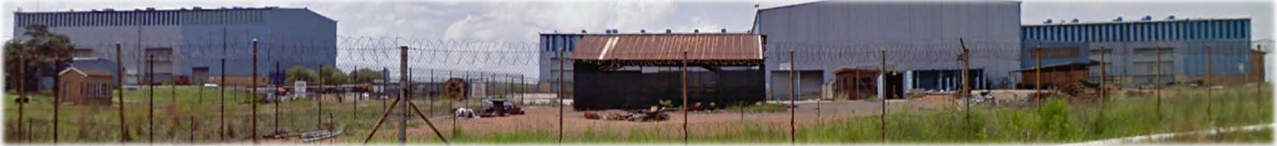
Figure 1 Dragline bucket repair workshop, ancillary workshops, and offices (Google 2010)
