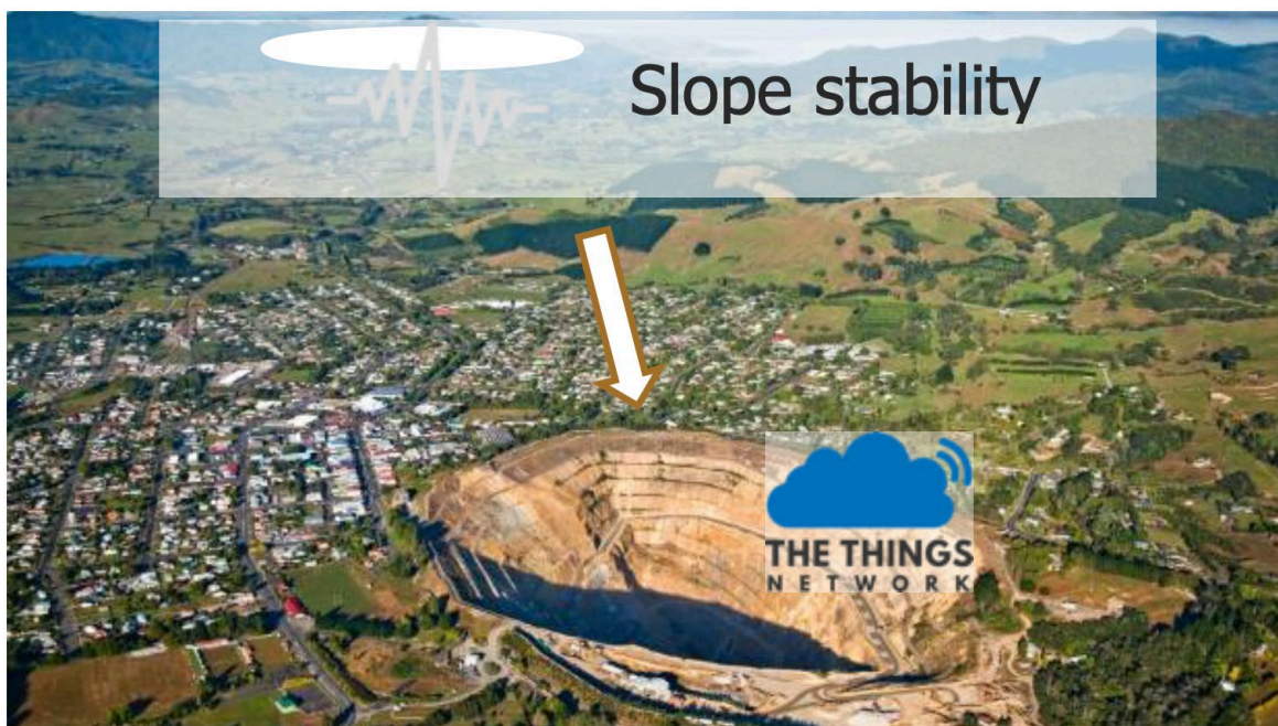
Figure 10 Slope stability monitors through Wi-Fi within an integrated network (Bowler 2018)
