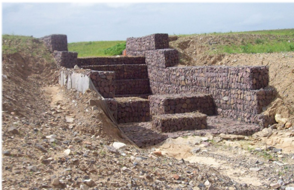
Figure 7 Soil loss: expose erosion control structures and imminent failure
