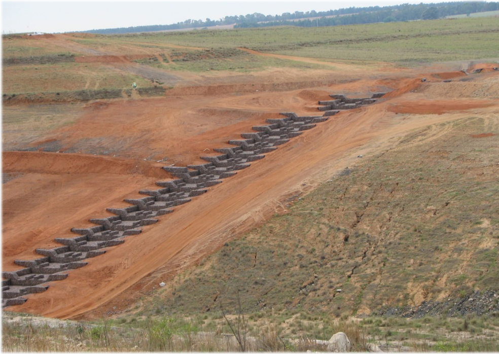
Figure 8 Gabion chute structure with exposed erosion gullies after first substantial rain event
