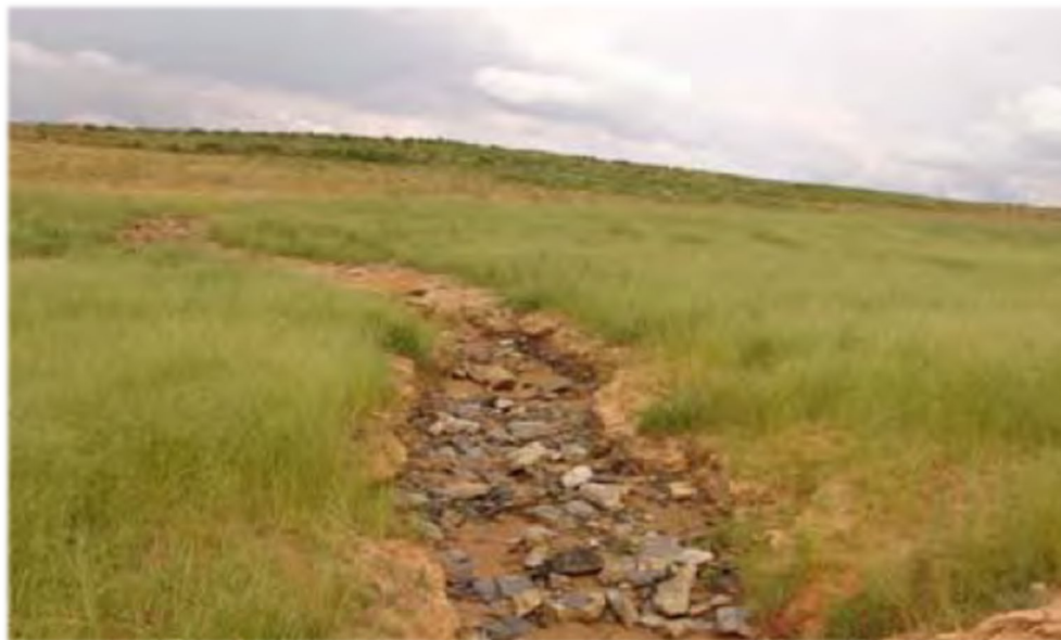
Figure 9 First rain season: exposure of spoil material
