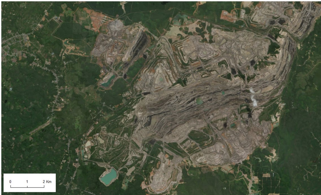
Figure 5 The Adaro complex: coal mines Wara, Tutupan, and Paringin in Indonesia. The risk profile of these mines contains multiple interplay of all ESG risks across the presented framework
