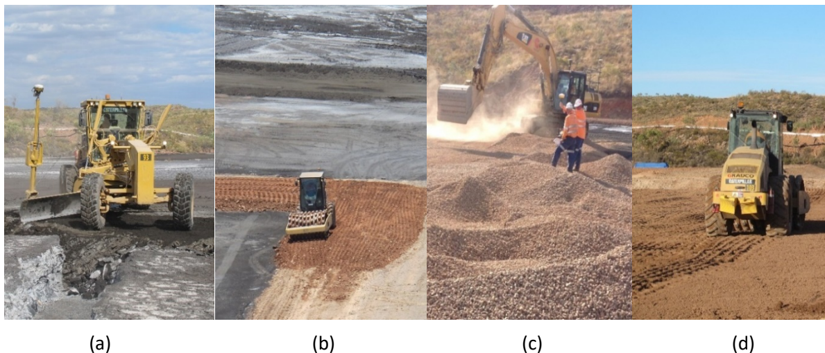
Figure 3 (a) Tailings beach preparation; (b) embankment construction; (c) capillary break placement; and, (d) reduced permeability layer (RPL) compaction (Defferrard & Rohde 2016)
