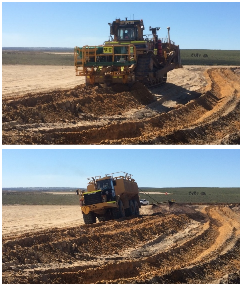
Figure 3 Rehabilitation practice in 2016 showing rip/mounding with seed and fertiliser broadcast (top) and application of dilute bitumen emulsion by water tanker from the unrippd surface (bottom)
