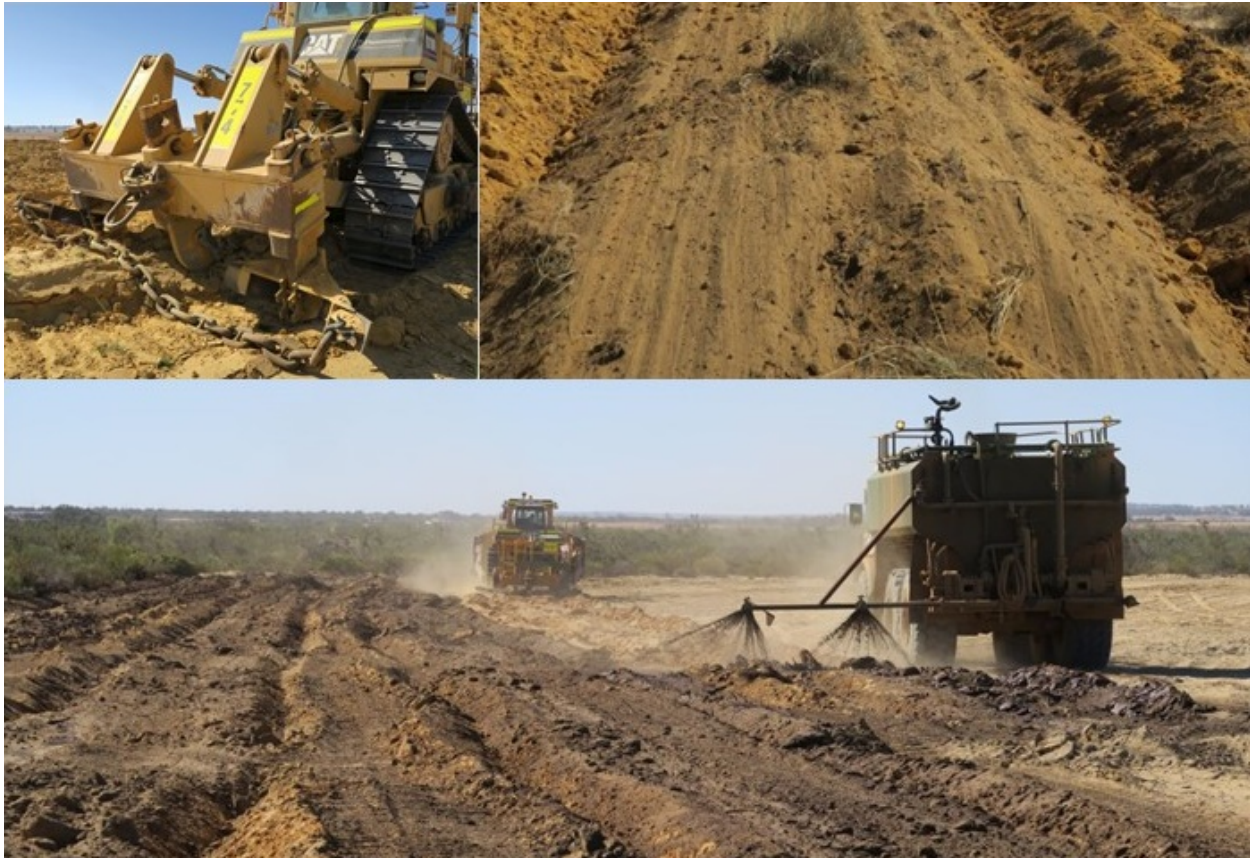
Figure 5 2017 rehabilitation rip/mound/chain equipment (top left) that created more 'flat areas' (top right), these were seeded and sprayed with dilute bitumen emulsion (bottom) similarly to 2016 rehabilitation
