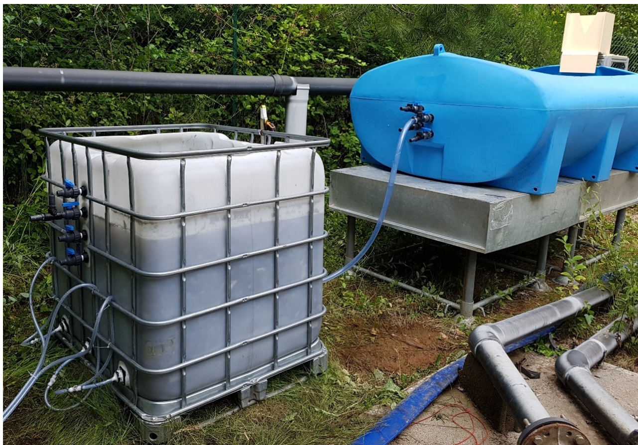
Figure 2 Picture of the pilot plant on site
