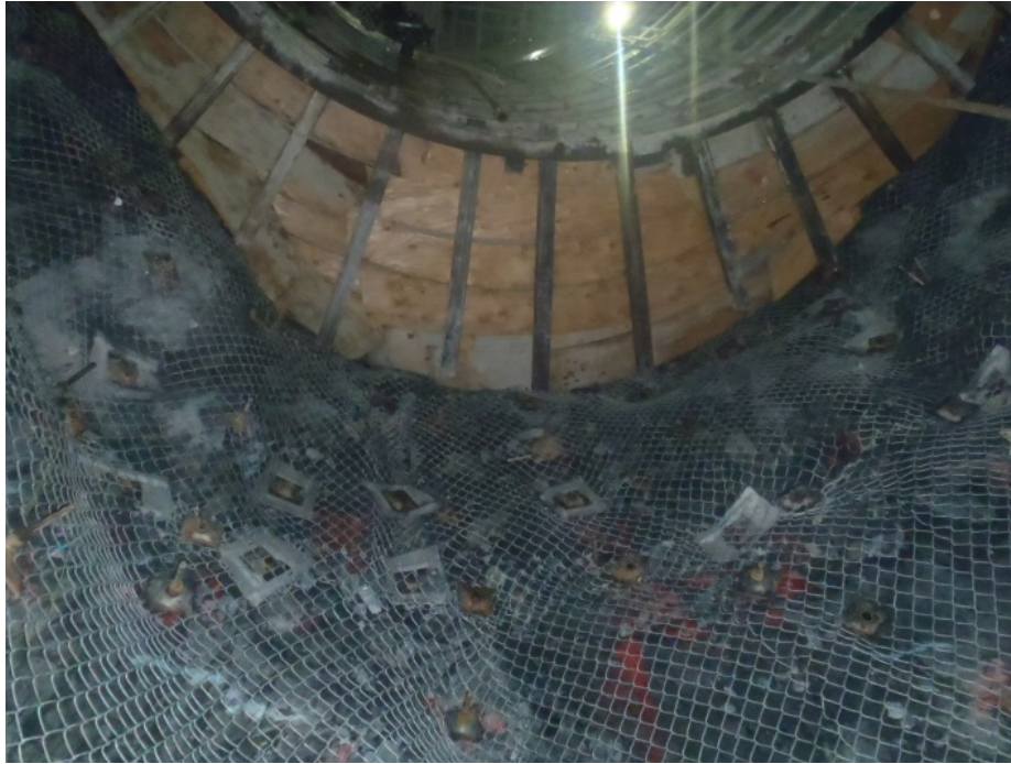
Figure 9 View up from shaft bottom showing the base of the liner after excavation of an elliptical shape for the shaft
