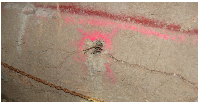
Figure 6 Cable bolt with plate sheared off and cable being pulled into the rock mass
