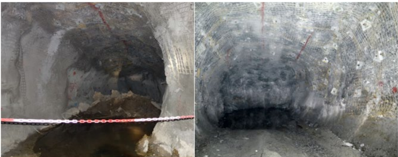
Figure 15 Much improved ground conditions using the new de-stress support scheme at South Deep
