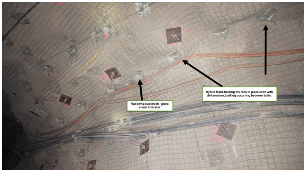
Figure 9 Image showing hybrid bolts being sucked into the rock mass
