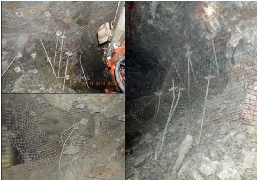
Figure 12 Ground support damage of the Garock hybrid bolts as pillars unravel around the highly fractured rock mass
