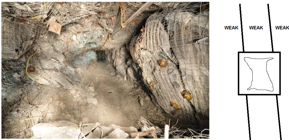
Figure 2 Late stage deformation in an ore drift entirely in ultramafics at Lapa (Mercier-Langevin & Wilson 2013)
