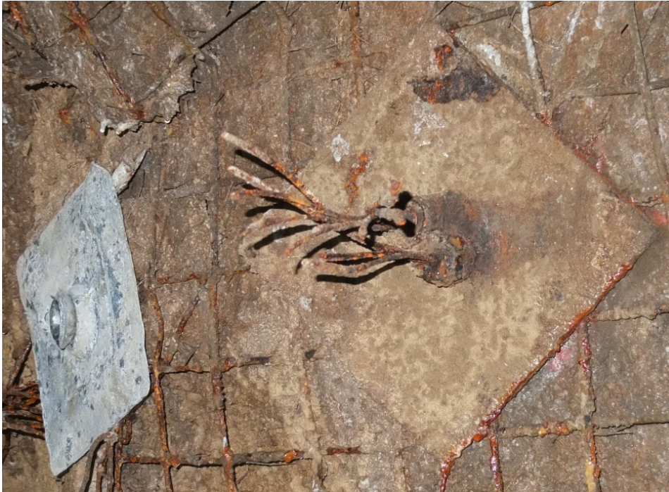
Figure 4 Example of different corrosion rates of ground support elements
