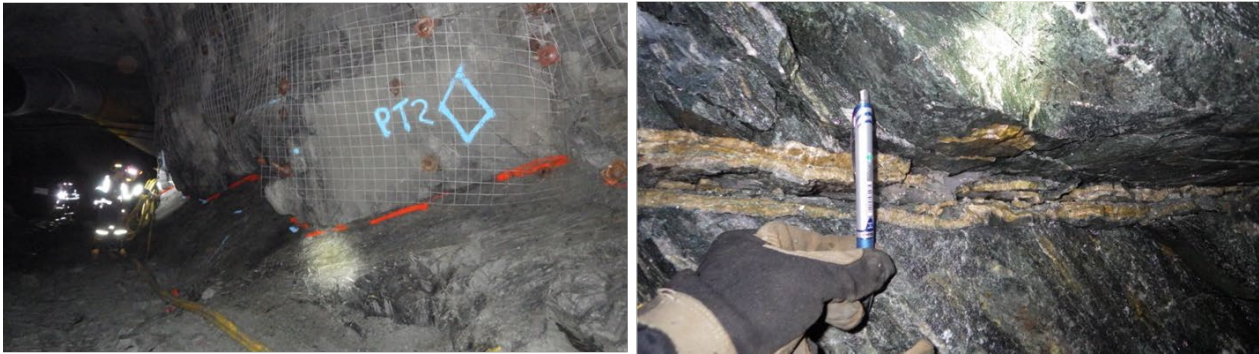
Figure 2 RM175 Fault with gouge and ice encountered during ramp development
