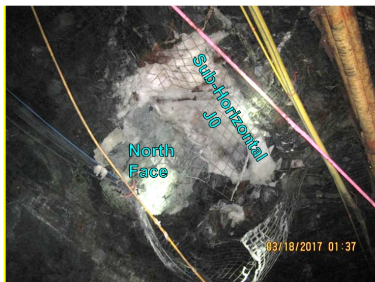
Figure 11 Ice formation along J0 behind the fallen block. The ice was visually estimated to be around 50 mm thick. Thinner ice (grey colour) was also noted along the 50° dipping joint surface on the north face of the block
