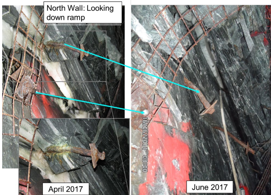
Figure 13 Ice build-up along the foliation (thick white bands) causing dilation and degradation of the wall
