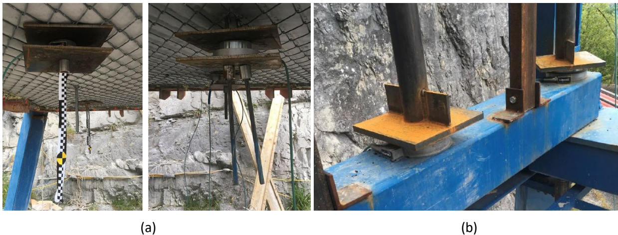
Figure 7 Load cell installation at (a) Solid bar and twin strand cable; (b) Abutment
