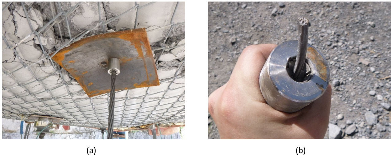
Figure 12 (a) Snapped cable bolt; (b) Twin cable bolt No. 2
