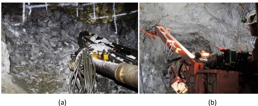
Figure 7 (a) Underground photo of a strainburst that occurred while drilling with a jumbo. In this situation the vein orientation changed drastically resulting in a stress concentration in the host rock; (b) Narrow vein boom-bolter in operation in a 3.3 × 3.3 m heading. The introduction of these units means a reduction in worker exposure (versus handheld bolting)
