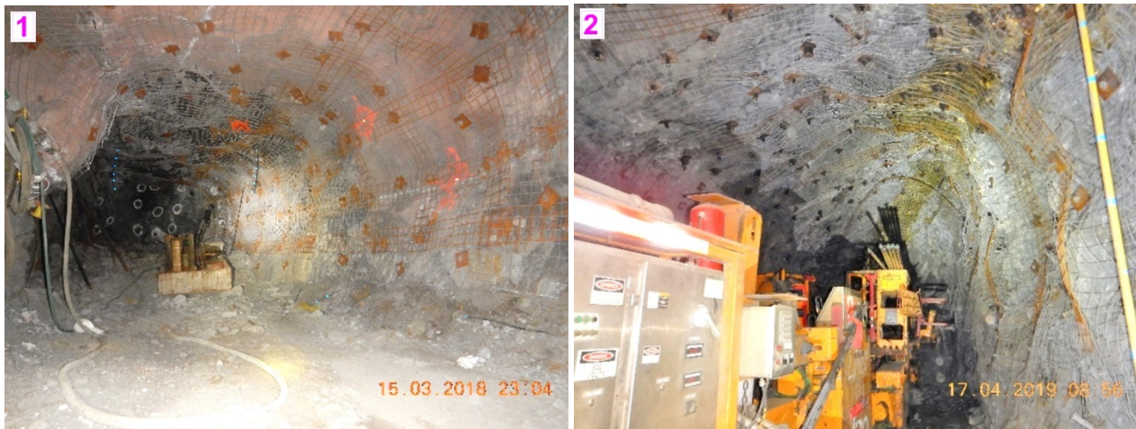
Figure 11 Underground photos corresponding to Figure 10 labels. (1 left) under-cut-and-fill heading with dynamic support (cross-straps) installed on potentially high stress right wall. Pink shotcrete is a fast-setting/high strength blend; (2 right) overhand cut-and-fill heading showing ground conditions and support installed on potentially high stress back and right wall (2.4 m/3.5 m yielding inflatables)
