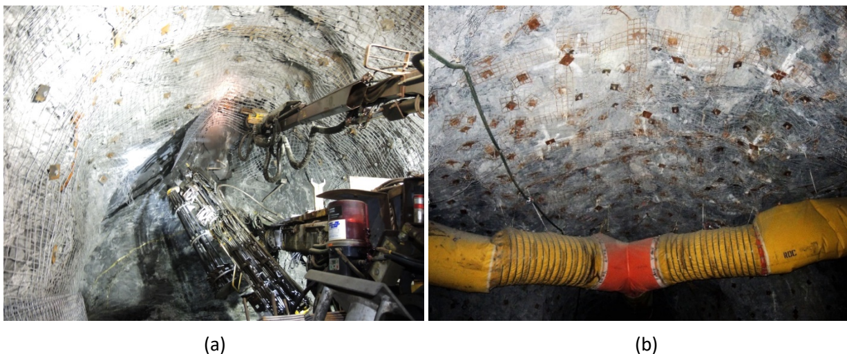
Figure 8 (a) Development boom-bolter in operation in a high stress development heading; (b) Underground photo showing ground condition encountered on 5950 level (notable rock bulking). The four-way intersection was seismically active while excavating. Primary back support consisted of 2.4 m resin-grouted dynamic bolts supplemented with 3.6 m yielding inflatables and straps in-cycle. Once excavated 5.5 m twin plated cable bolts were installed
