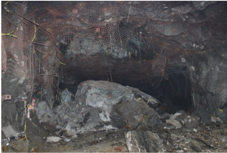
Figure 1 Fall of ground in a drawpoint caused by reduction of support system capacity related to corrosion
