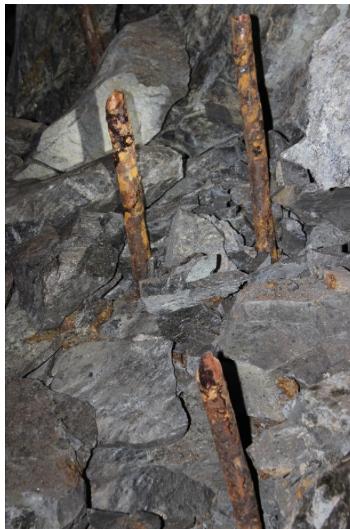
Figure 2 Heavily corroded inflatable bolts attributed to a fall of ground
