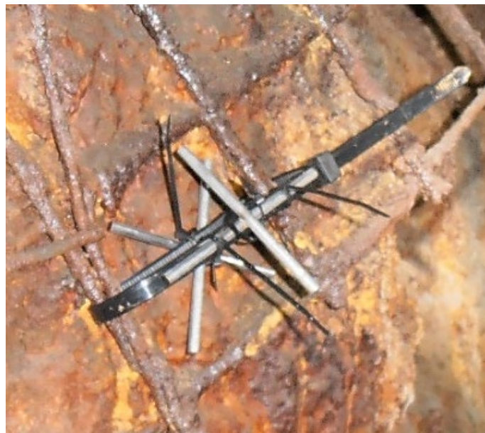
Figure 3 Welded wire mesh coupons in the field
