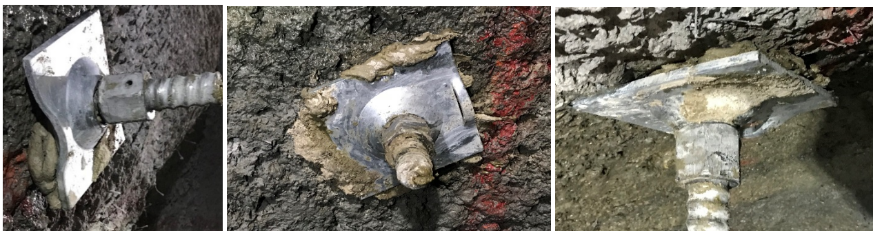
Figure 14 Installation of multiple R32 MPA bolt using the J-Lok P resin injection
