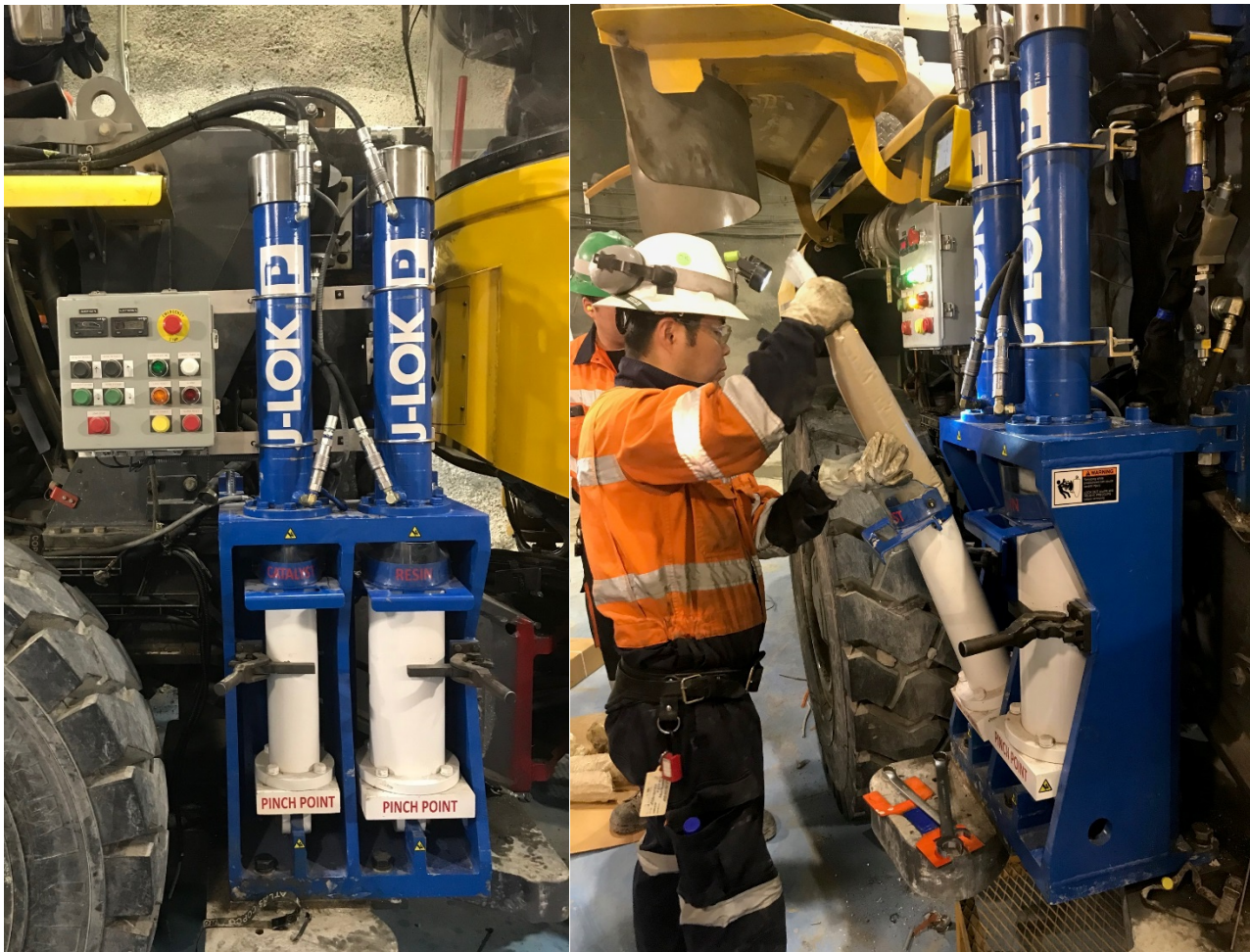
Figure 2 J-Lok P resin loading cylinders and catalyst (smaller 7 kg white bag) being loaded into injection tube
