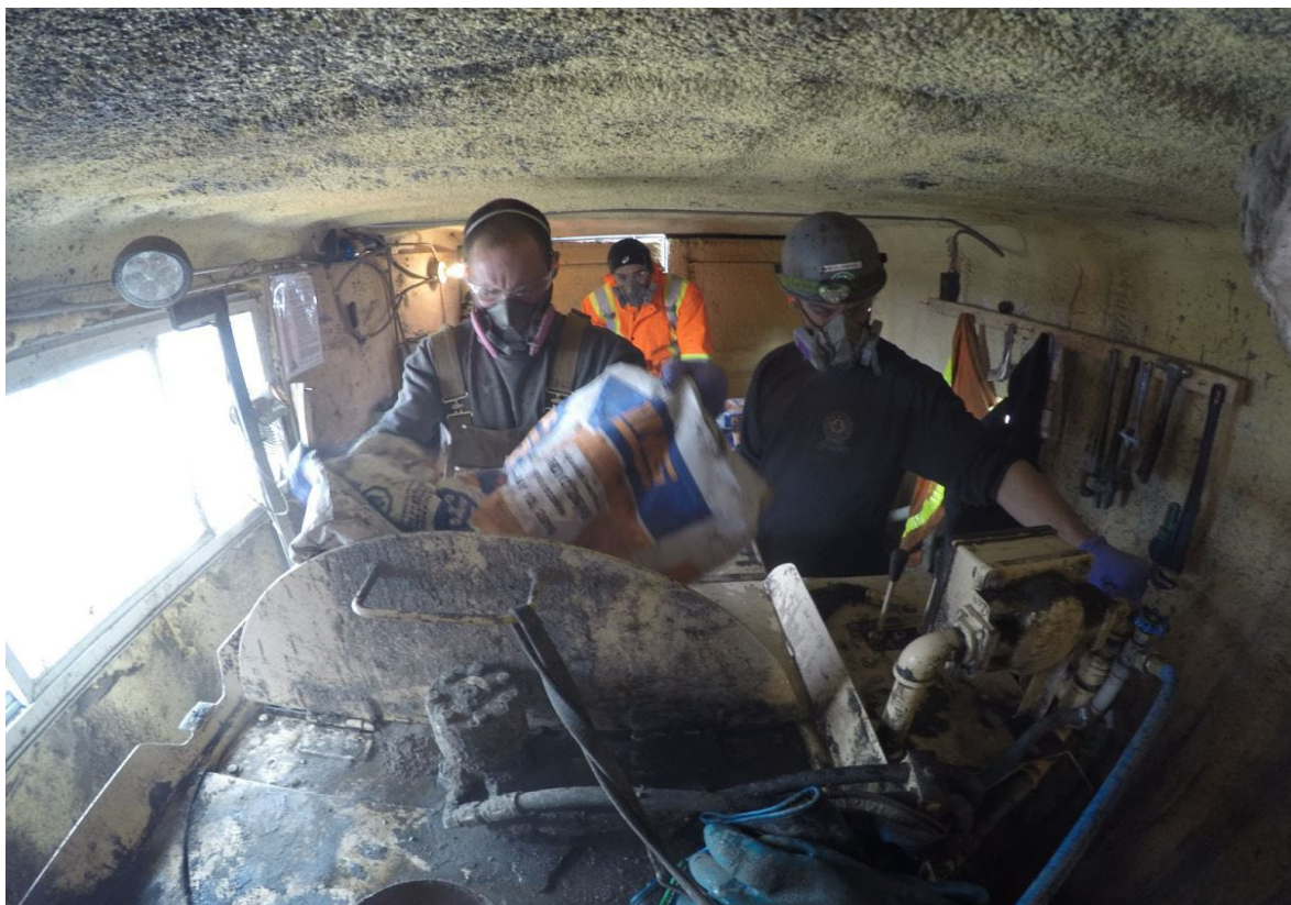
Figure 1 Grout batch plant stored in insulated and heated container
