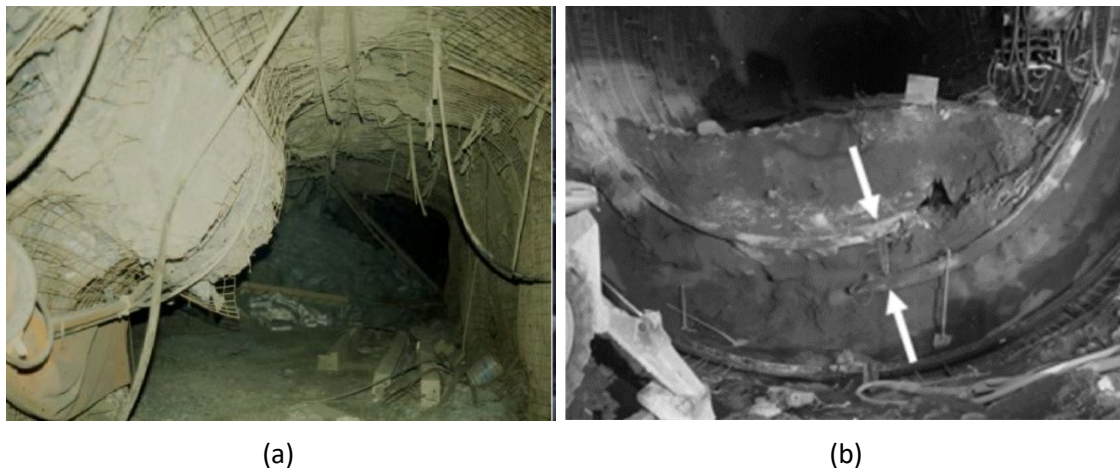
Figure 1 (a) Support system damaged by rockburst (Kaiser & Cai 2013); (b) Sheared-off steel arch caused by squeezing behaviour (Rehbock-Sander & Jesel 2018)
