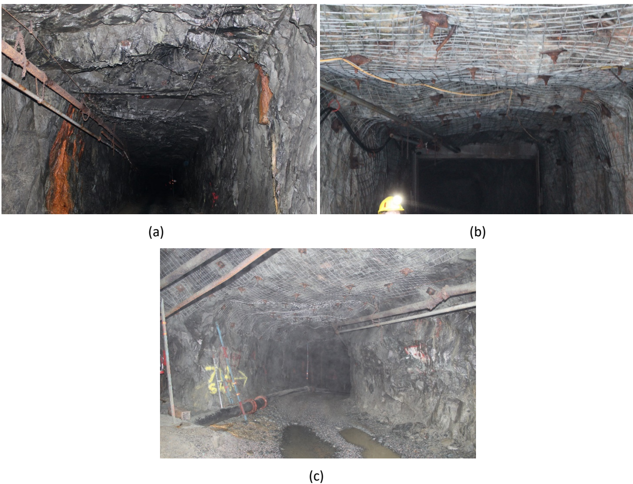
Figure 5 (a) Spot bolting ground support; (b) Systematic bolting and welded wire mesh ground support; (c) Systematic bolting and welded wire with longer bolts for intersection support
