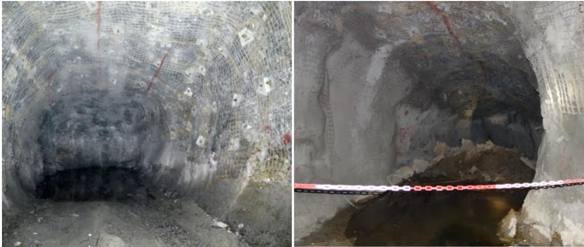
Figure 11a. HPS development with bolts and mesh
