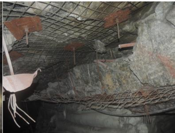
Figure 8b. Opening of bedding planes in LPS
