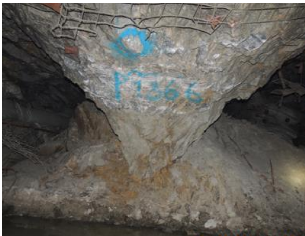
Figure 8a. Deteriorated crush pillar in LPS
