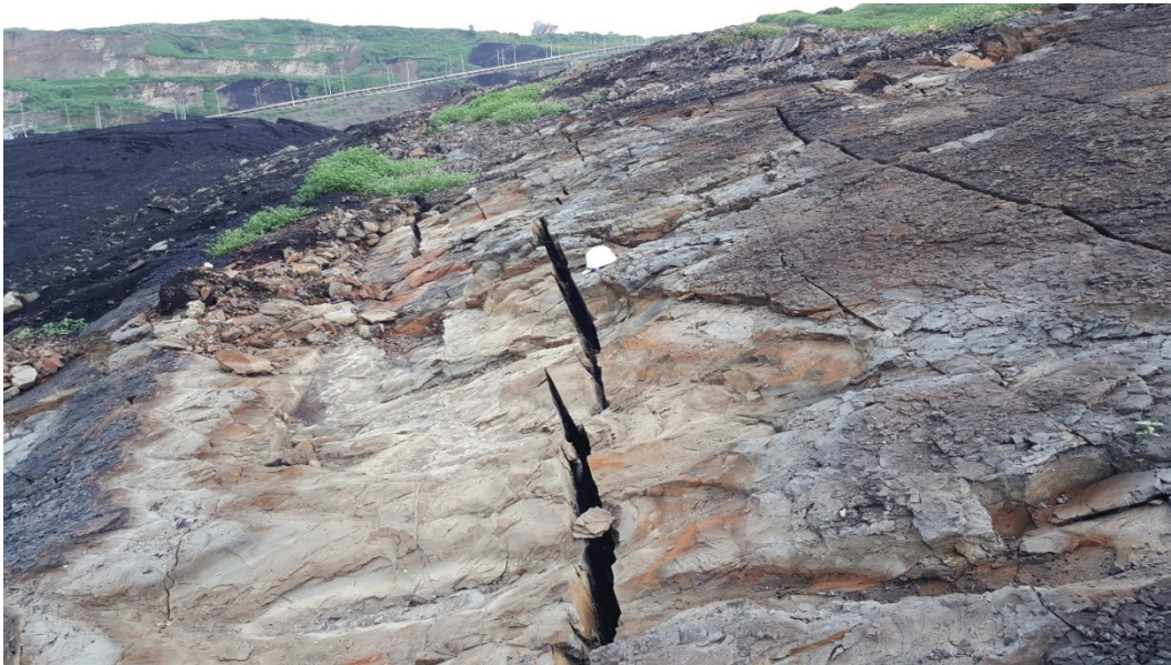
Figure 19 A typical footwall showing aperture development on joints in an advanced stage of movement
