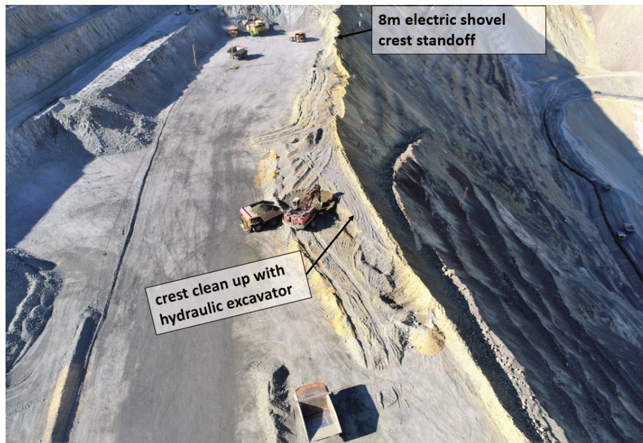
Figure 15 Crest mining using hydraulic shovel where crest stand-off is required for rope shovel
