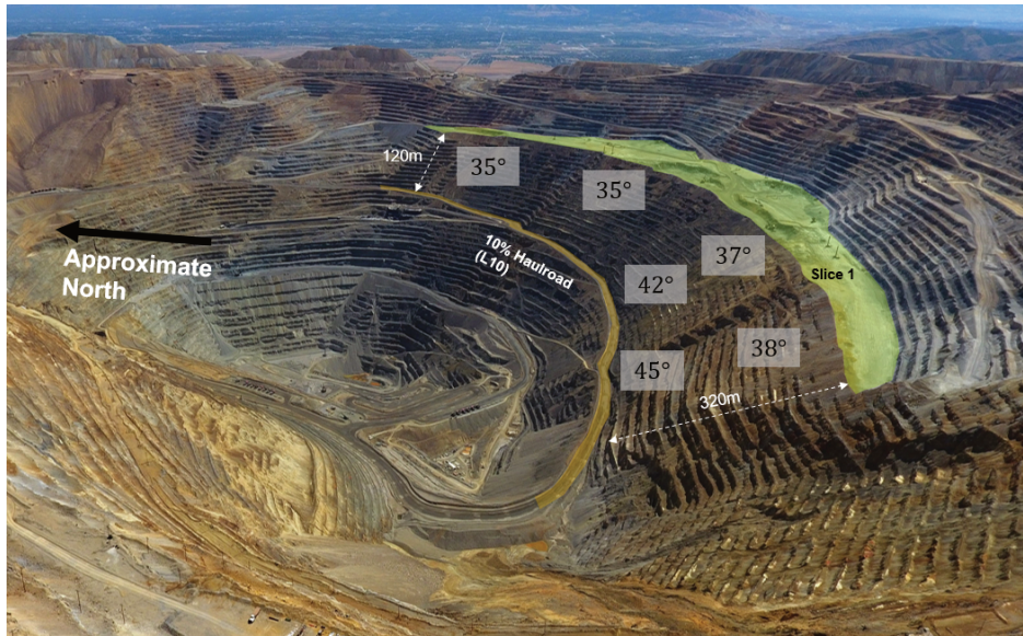
Figure 3 South wall showing slope height and inter-ramp angles
