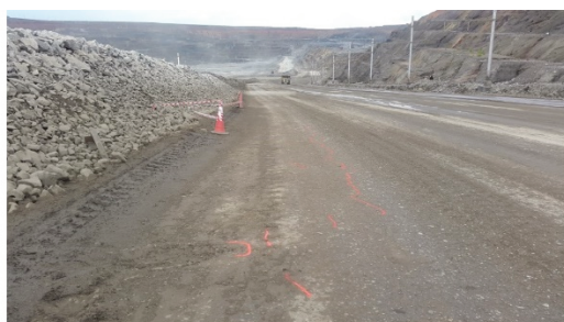
04 December 2017 (tension crack development)
