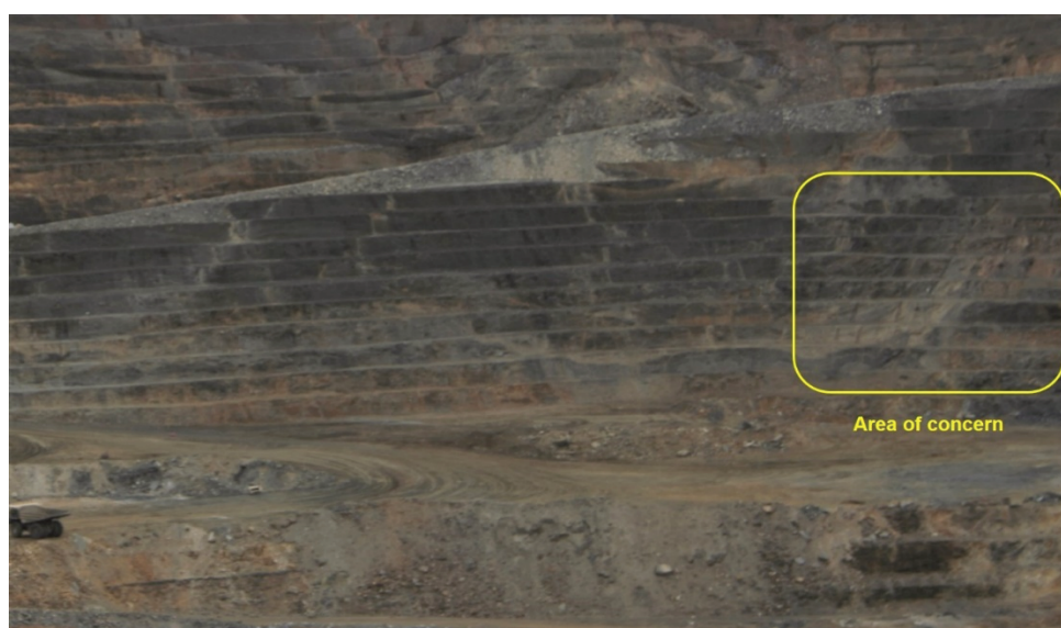
Figure 19 Continued weathering of exposed walls in Main 12 North-East (November 2017)
