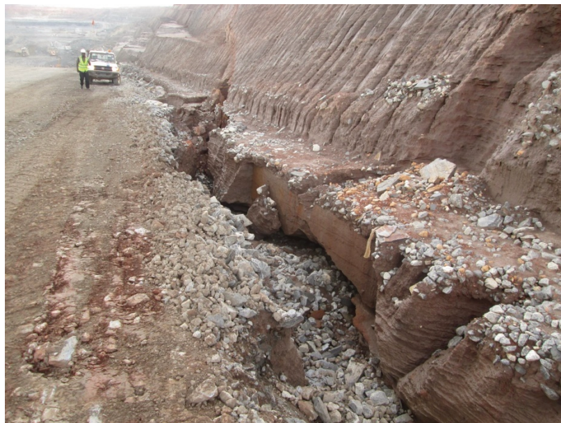
Figure 7 Sinkholes observed on Main 10 ramp during early 2015
