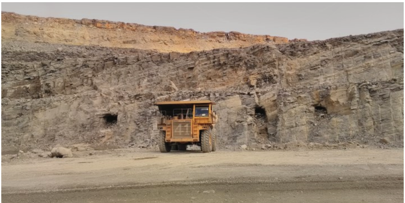
Figure 2 Tunnels intersected during surface mining
