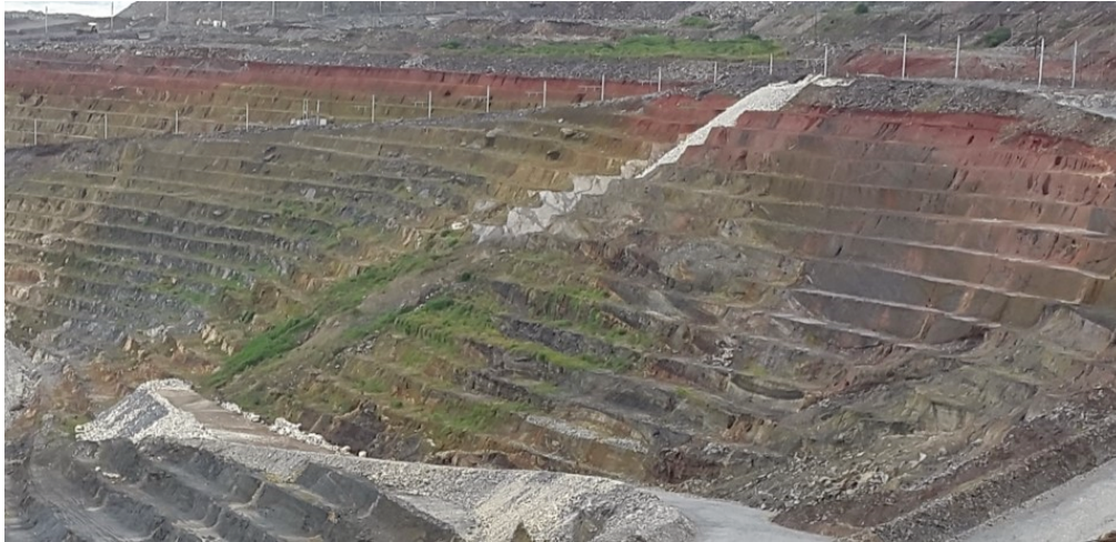
Figure 18 Backfilled wedge failure footprint and constructed abutment
