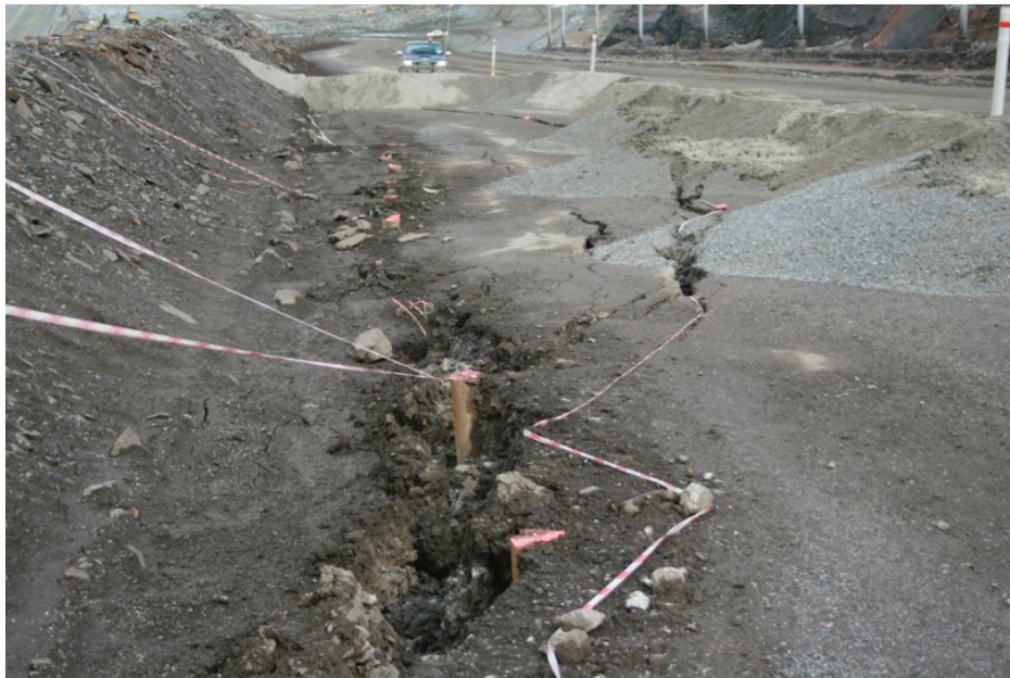
Figure 10 Six-metre long piles exposed along tension cracks on the ramp in February 2016
