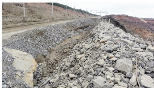
09 March 2018 (0.6 m vertical displacement along tension crack)
