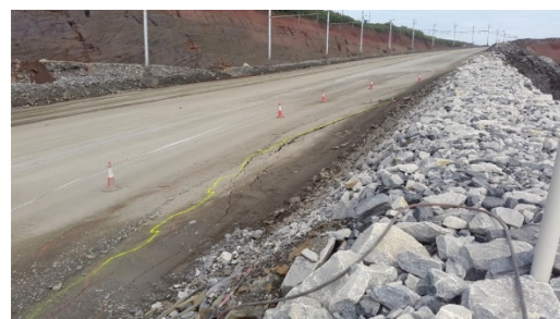
01 February 2018 (vertical displacement along tension crack)
