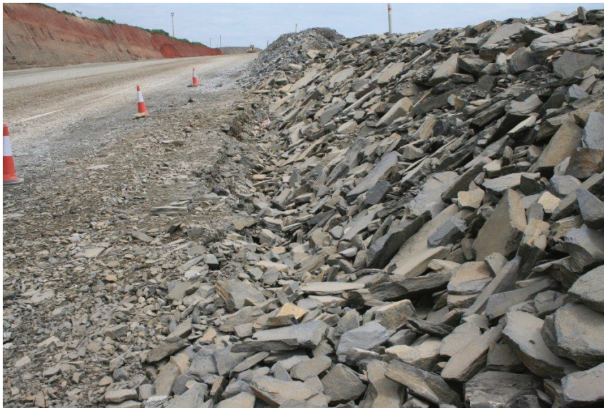
Figure 9 Slumping of the windrow on the M10 trolley ramp
