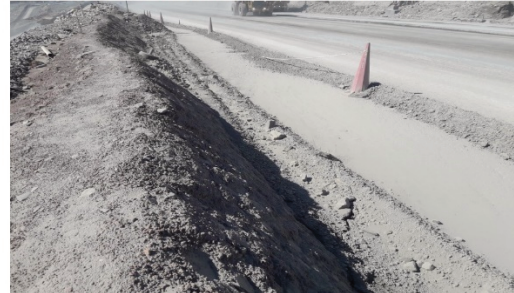
22 March 2019 (sloughing of windrow over the wall)
