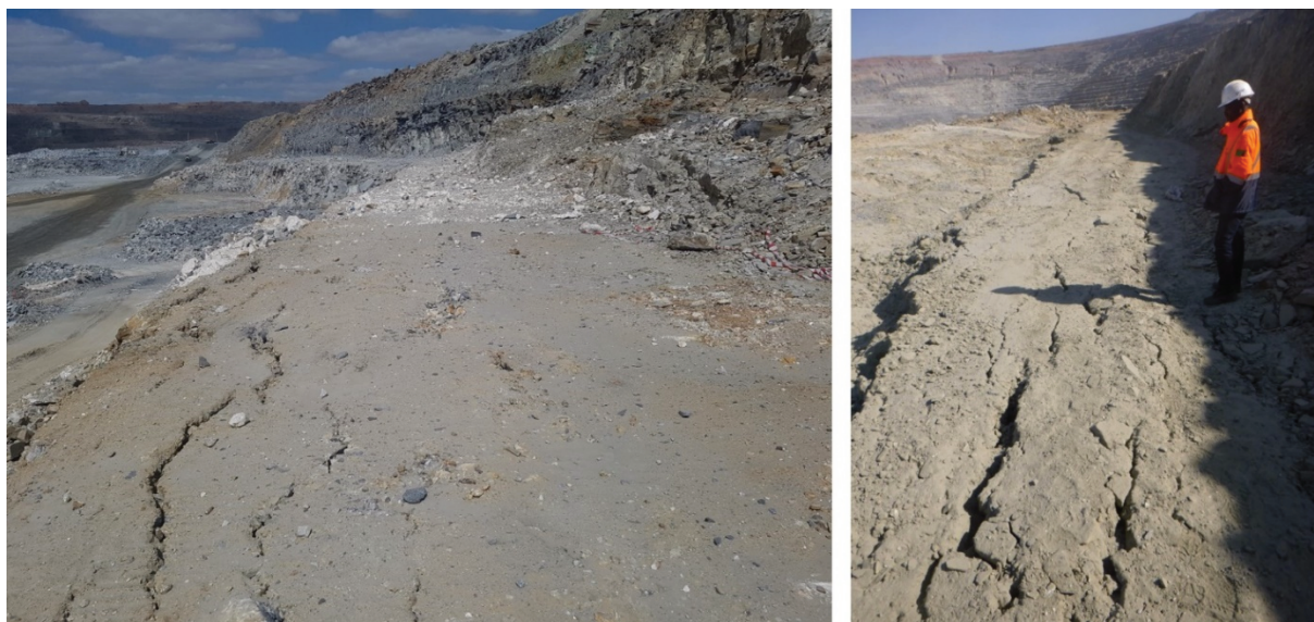
Figure 21 Examples of overbreak from the presplit blast
