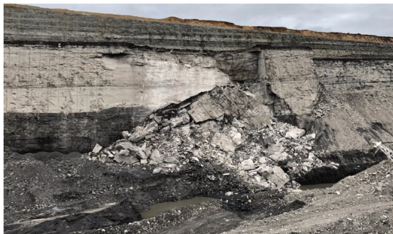
Figure 9 Post-failure of the highwall after the trial was completed
