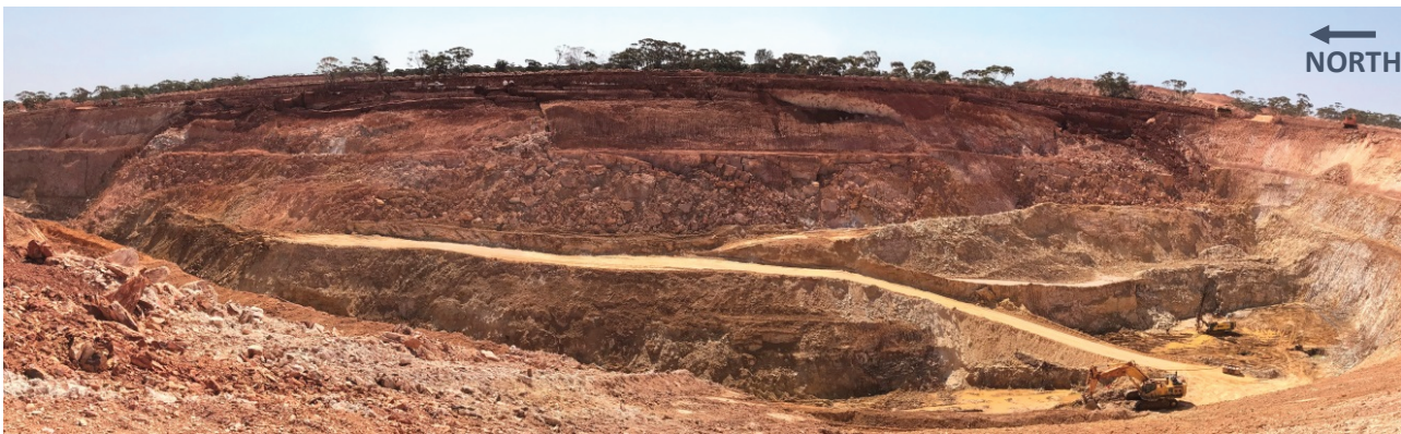
Figure 5 Eastern pit wall before slope unloading, showing the large-scale instability and strategic buttressing material (midground). Pit wall is 40 m in height
