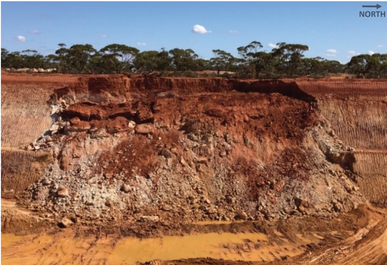
Figure 4 Observed instability along the western pit wall. Instability is 20 m in height
