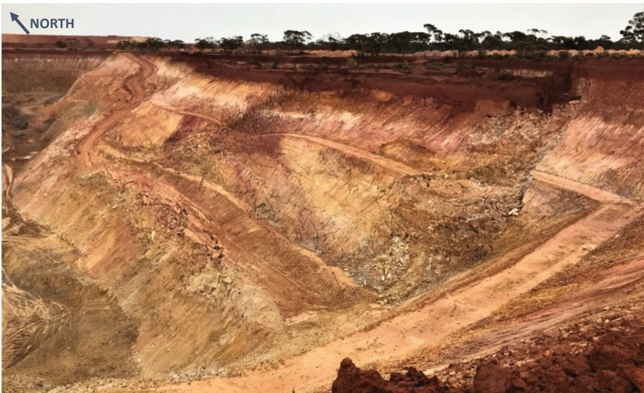
Figure 10 Eastern pit wall instability at the completion of mining. Note the dislocation of benches and deformation of the haul road
