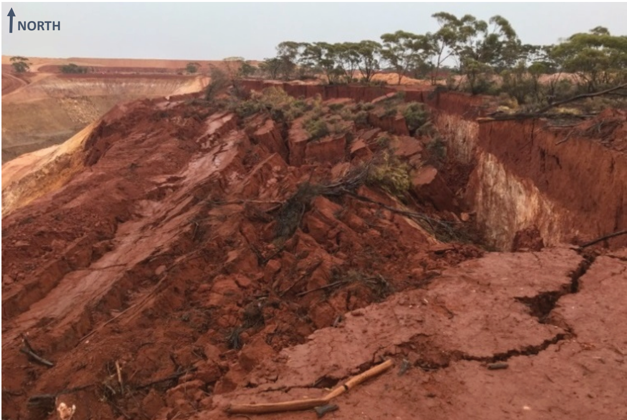
Figure 9 Head-scarp of the eastern pit wall instability at the completion of mining
