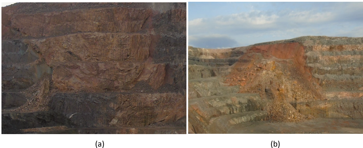
Figure 1 Southeast highwall: (a) Pre-failure (2018-07-02); (b) Post-Failure (2018-07-05)
