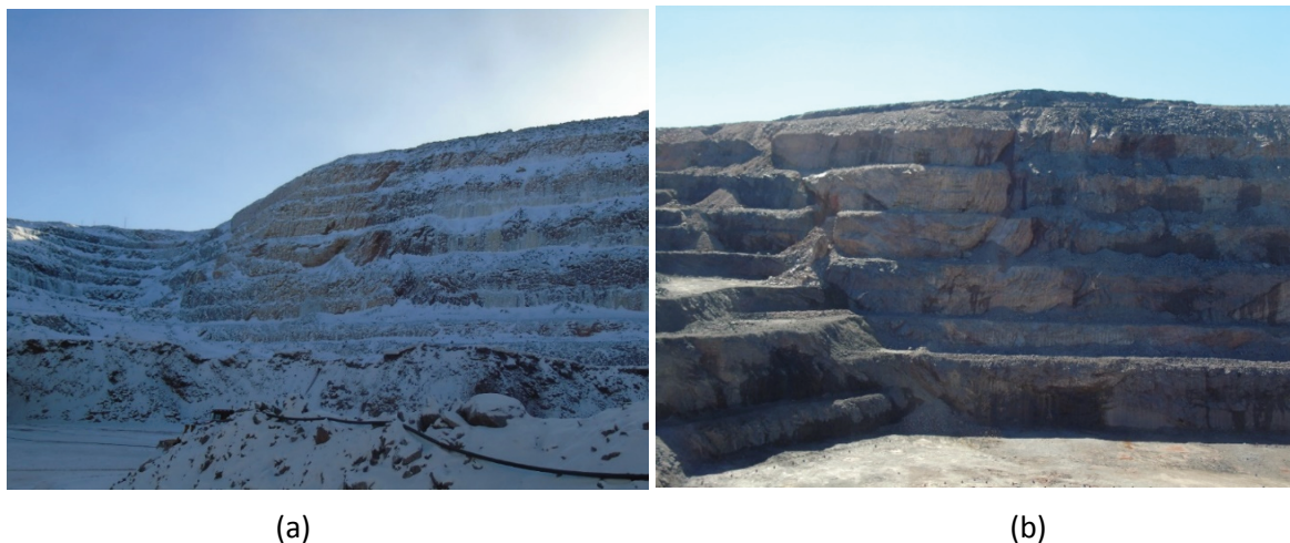
Figure 4 (a) Ice formation due to groundwater drainage surrounding the failure mass; (b) Post-thaw conditions of the slope surrounding the failure mass
