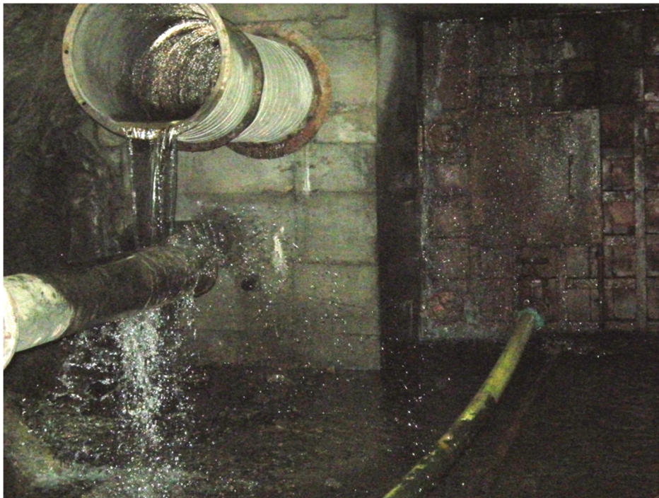
Figure 4 Example of an ageing bulkhead where the water level has risen past the drainage valve
