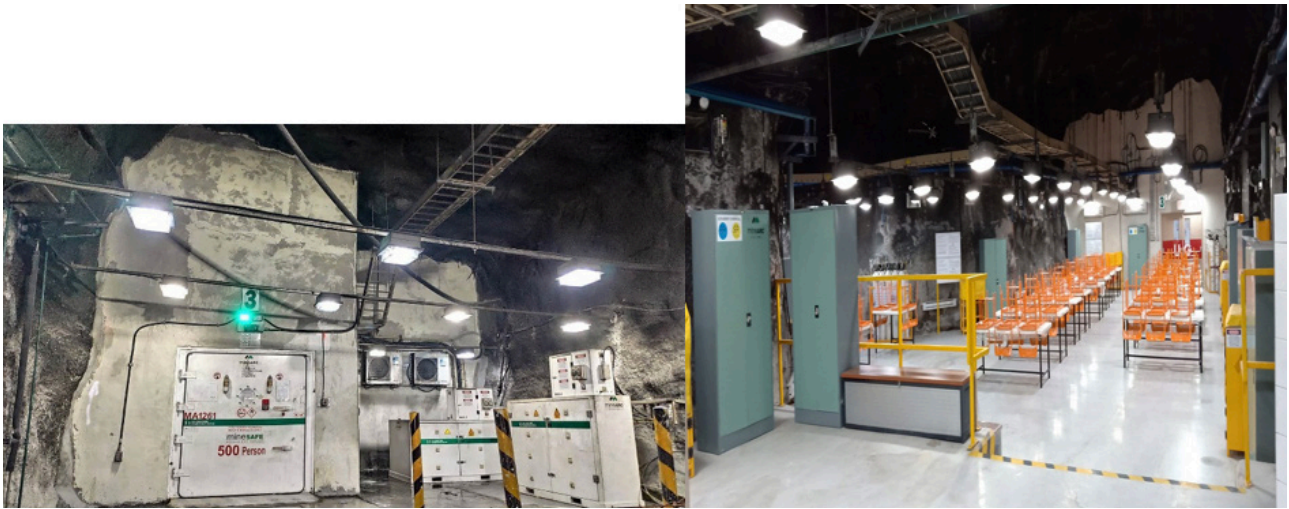
Figure 7 GBC 500-man permanent refuge chamber, showing one external entrance and one section of the interior of the chamber
