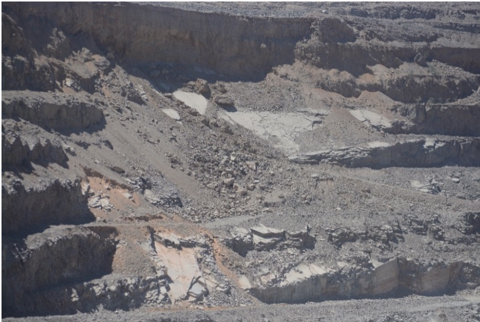
Figure 4 Three-bench failure in the eastern side of the pit
