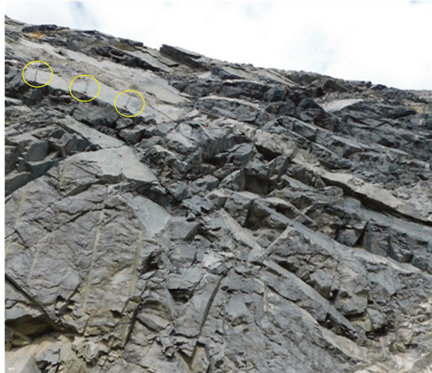
Figure 4 Unstable blocks on pit wall supported with grouted cable bolts (shown by yellow circles)
