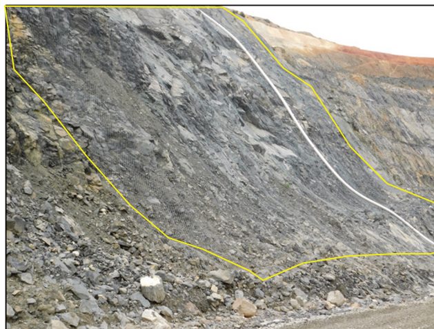
Figure 3 Pit wall with a drape mesh controlling rockfall trajectory
