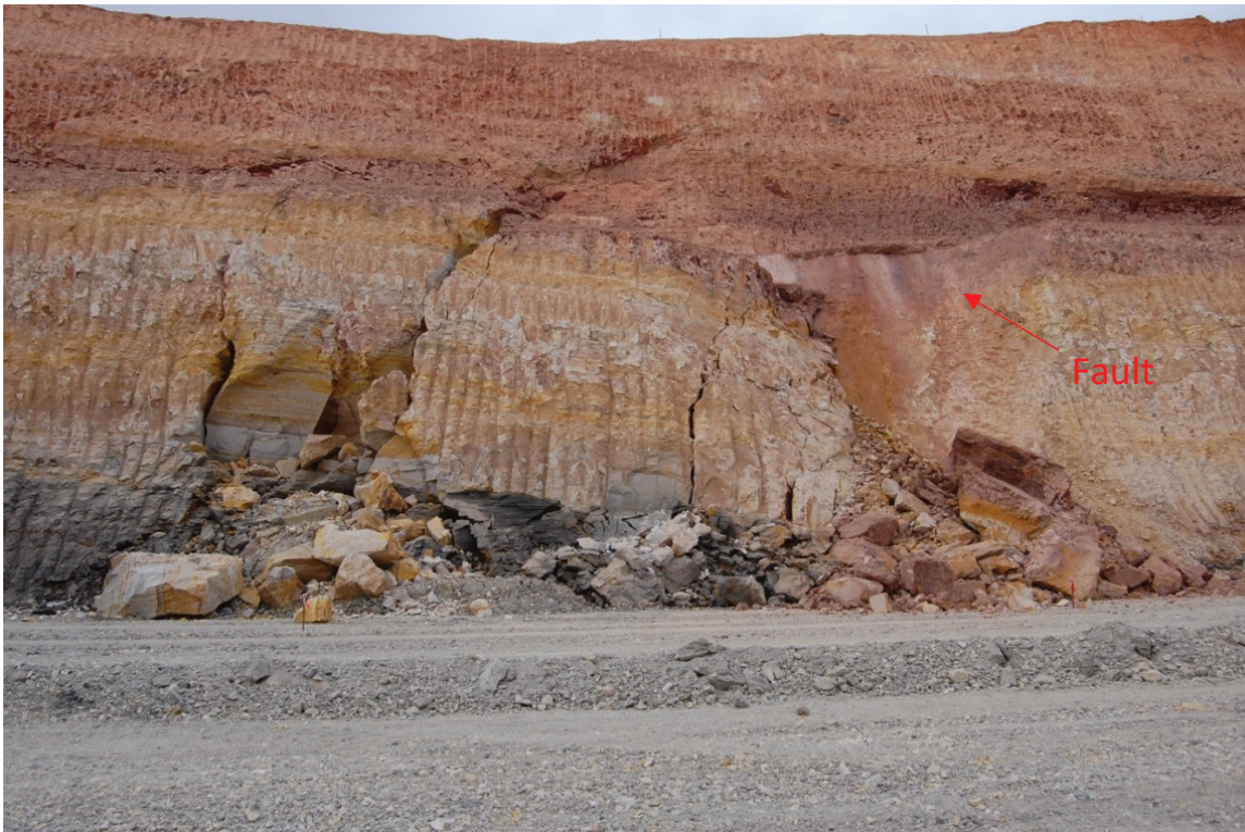
Figure 17 Small one-sided wedge, fault-bound on one side with failure through rock mass on the other. This is one bench high (15 m)
