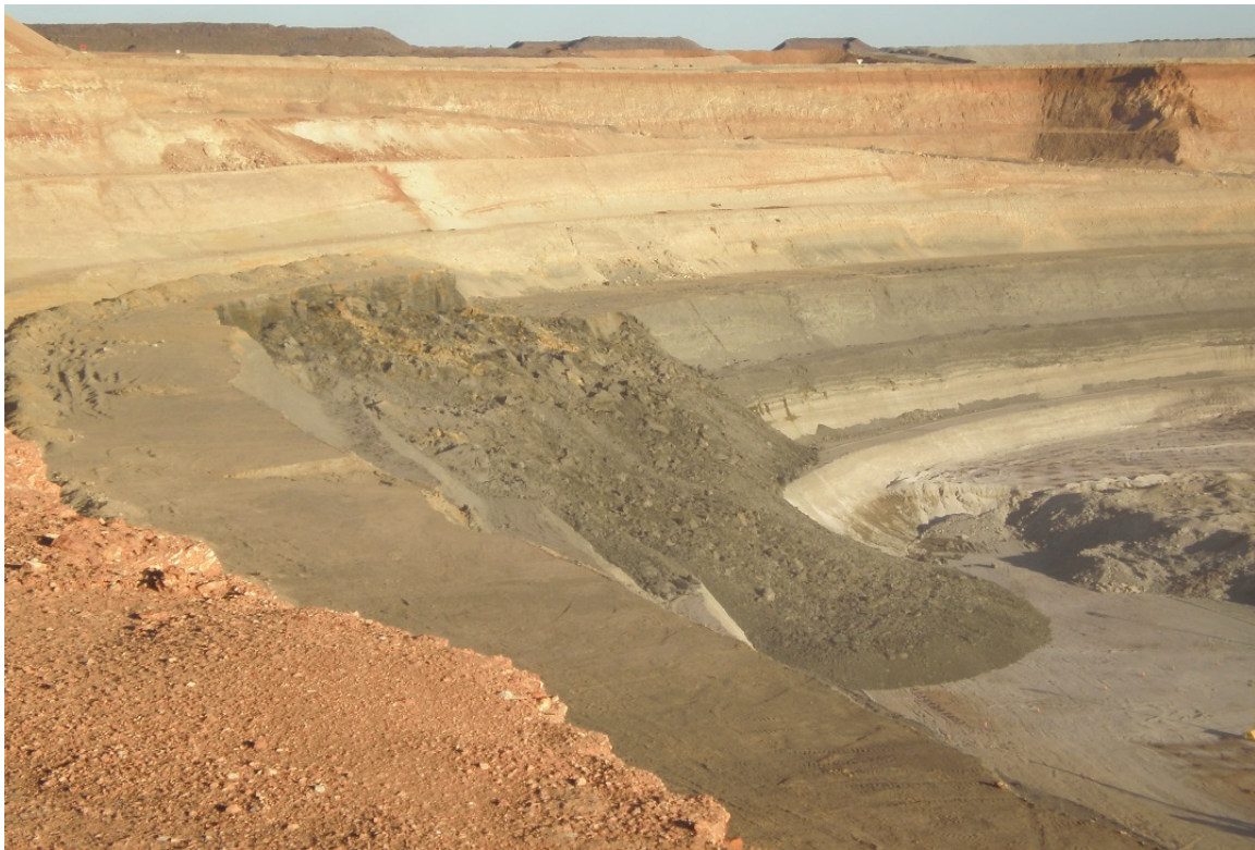
Figure 19 Medium-sized failure showing runout over the working surface. This is about 50 m high
