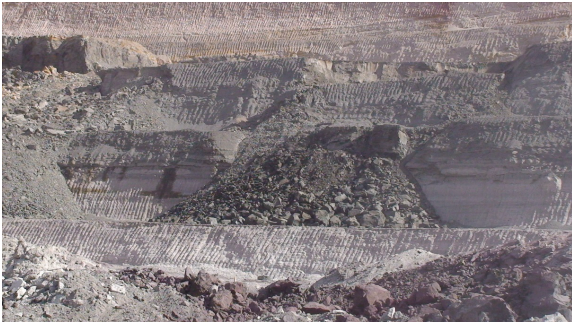
Figure 18 Small non-daylighting wedge, where two faults define a block with a hinge line that is steeper than the slope angles. Failure develops by sliding on bedding at the base. This is two benches high (30 m)
