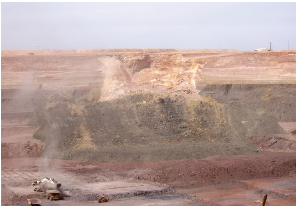
Figure 20 Larger-scale (>200,000 BCM) non-daylighting wedge over the inter-ramp scale with significant runout over the working floor
