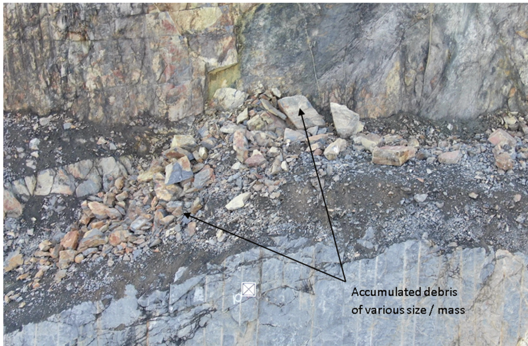
Figure 2 View facing source of rockfall and showing accumulated debris beneath
