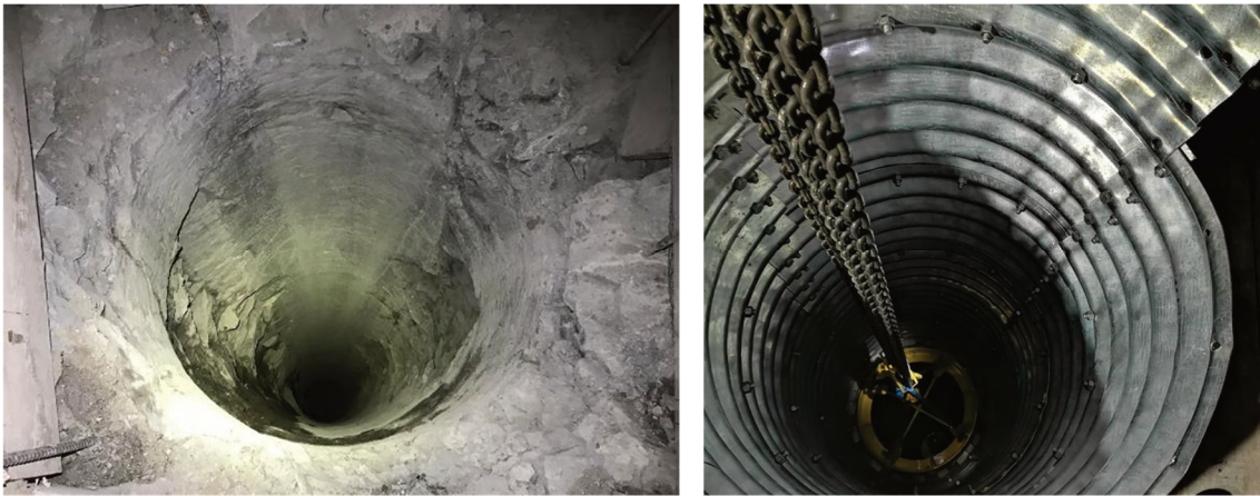
Figure 14 Ventilation shaft overbreak. Steel liners installation process to control future instability (Madrid 2020)
