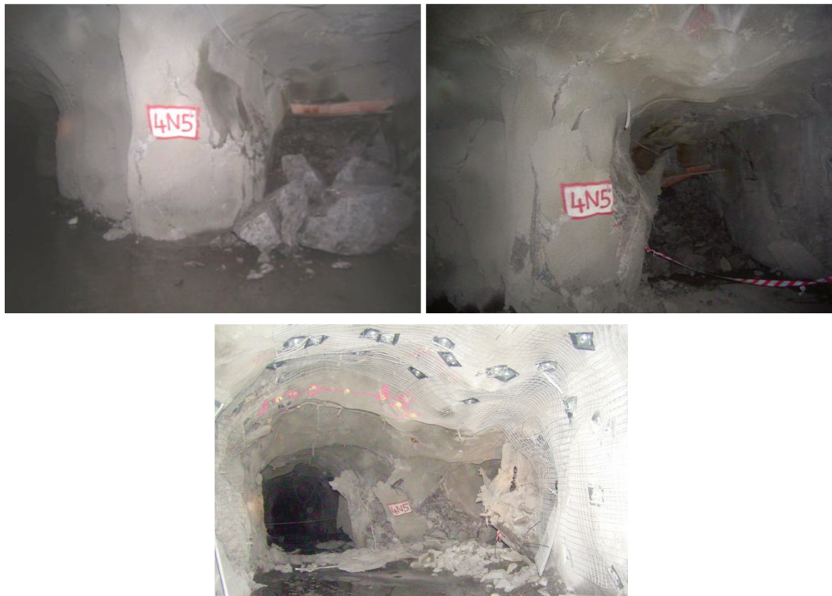
Figure 5 Progressive failure over three weeks of ED4–4N5 area
