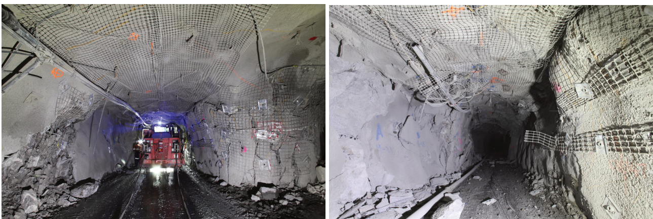
Figure 9 Deterioration in EDA during March 2015
