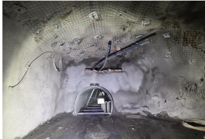
Figure 10 Western end of EDA plug with AS8 to the right
