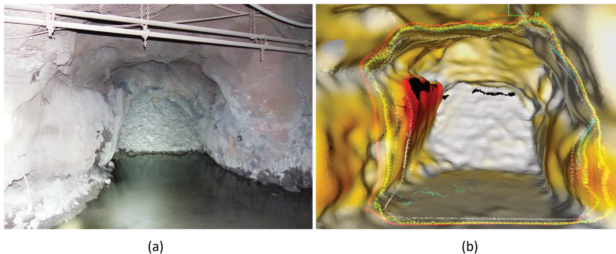
Figure 13 (a) Picture of F40N exceeding 4 mm/day; (b) Triangulation and point cloud cross-section overlaid to illustrate convergence over time (scale as noted in Figure 12)
