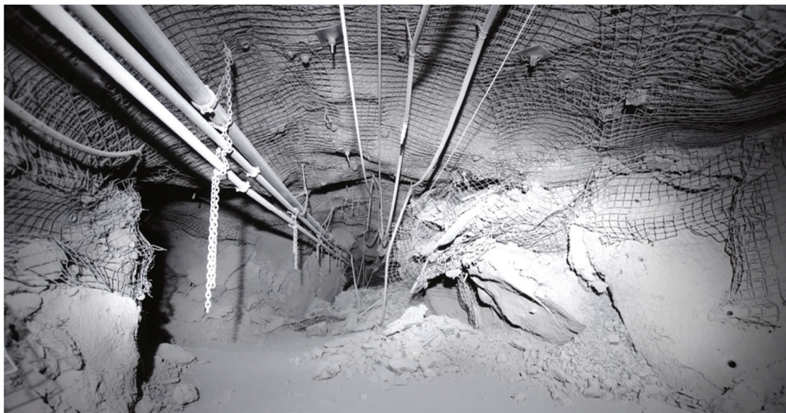
Figure 22 View looking down a late-stage converged extraction drive permanently closed post-production. Original 4.5 × 4.5 m drift converged to less than 2.0 × 2.0 m in several areas. Observations show yielded and toppling pillars with an observed flat looking back profile with intact ground support and very little to no shotcrete cracking, aligning with the MPBX data observed in Figure 21
