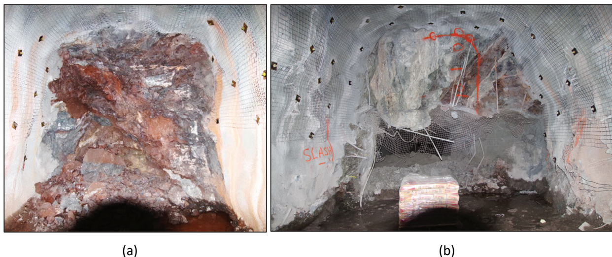
Figure 3 (a) Example of alteration effects on the BXF–diorite contact resulting in RMR < 37 , and the rock mass from the face sloughing after scaling; (b) Extraction drive undergoing rehabilitation due to high levels of convergence in similar faulted and altered rock mass
