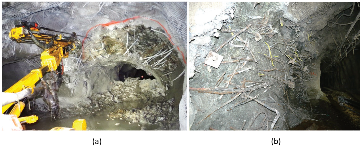
Figure 15 (a) Drilling the redevelopment face; (b) Example of old/damaged bolts from redevelopment, requiring removal prior to new support
