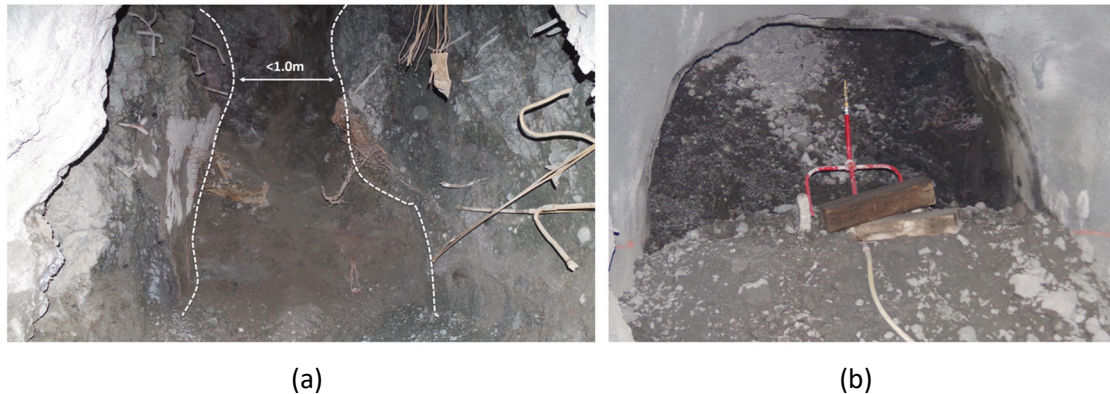
Figure 18 (a) Compaction beyond the brow observed after redevelopment of a fully converged drawpoint, the dashed lines represent converged walls within the drawpoint (originally 4.2 m wide); (b) Water sprayer used to assist with loosening the compaction to re-establish the flow of the ore column
