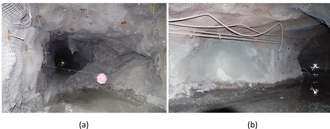
Figure 10 View of two separate areas of extraction drive with high convergence rates (>4 mm/day). (a) A drawpoint without concrete, resulting in extraction drive deformation; (b) Filled with oversized material and concrete resulting in a more stable strikedrive
