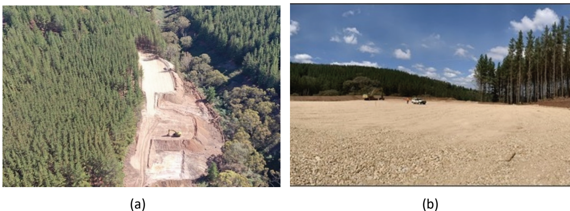
Figure 5 (a) Drill pad construction in progress (February 2020); (b) Completed drill pad (March 2020)
