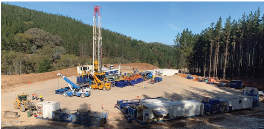
Figure 6 Drill rig setting up on first collar at North Drill Pad (April 2020)
