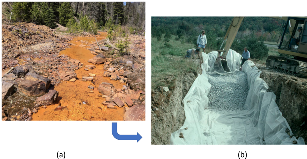
Figure 1 (a) AMD of an abandoned mine in the USA (photo courtesy of R Williams); (b) Open carbonate channel with limestone during construction (photo: J Skouson)
