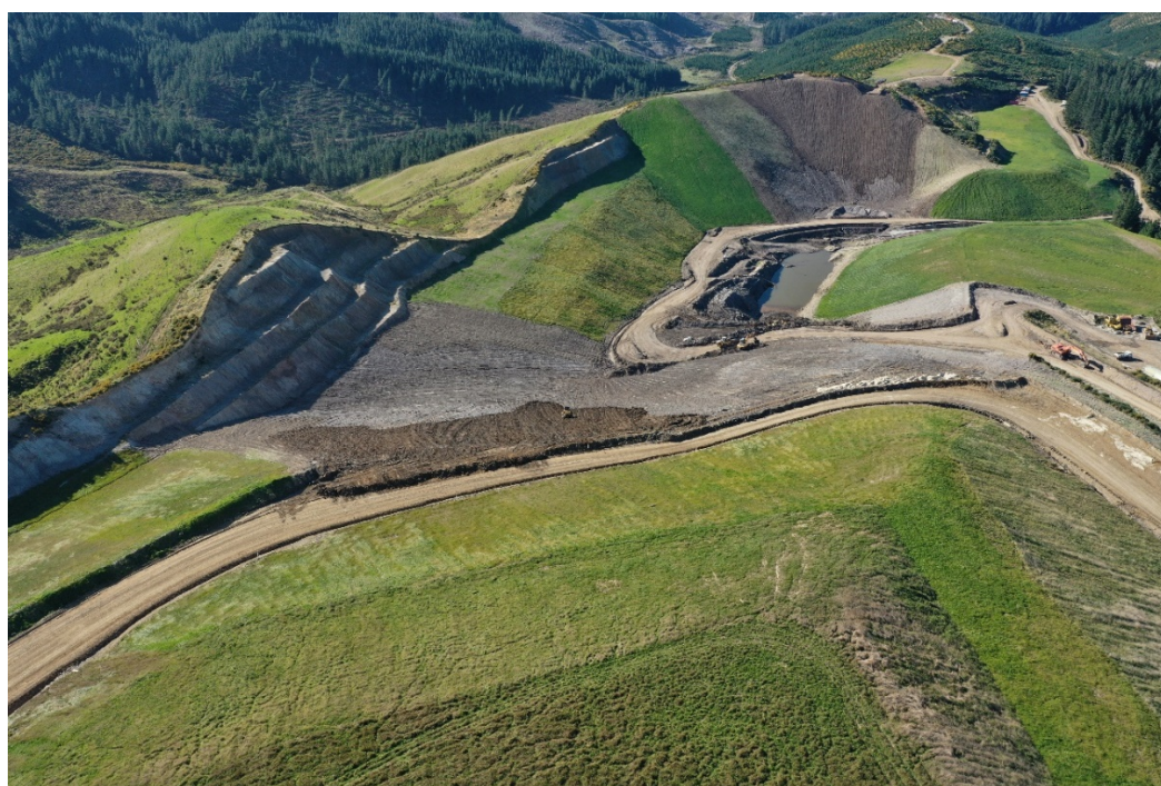
Figure 12 Site view showing final rehabilitation efforts and the N02 Pit Pond area
