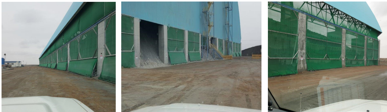
Figure 4 Installed dust curtains at the coarse ore storage facility, from west, front, and east sides
