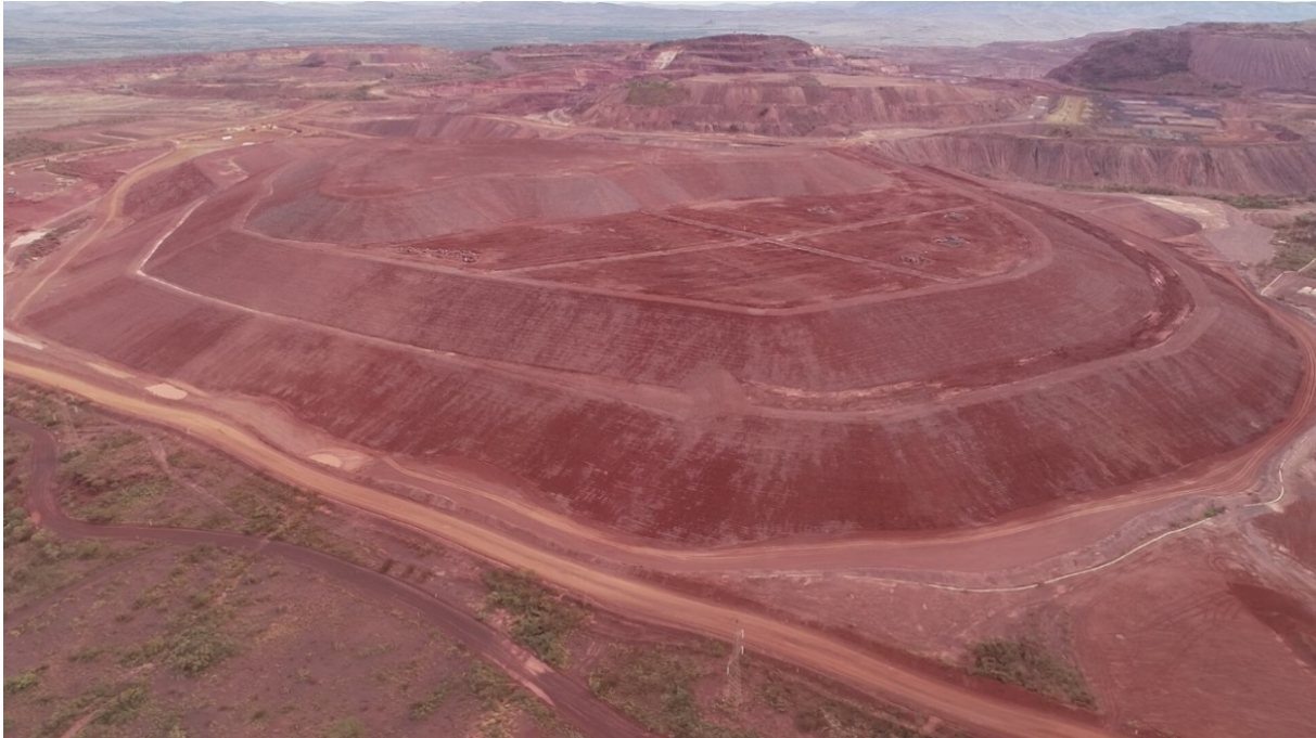
Figure 7 Overview of the NEBC waste dump earthwork completion, January 2022
