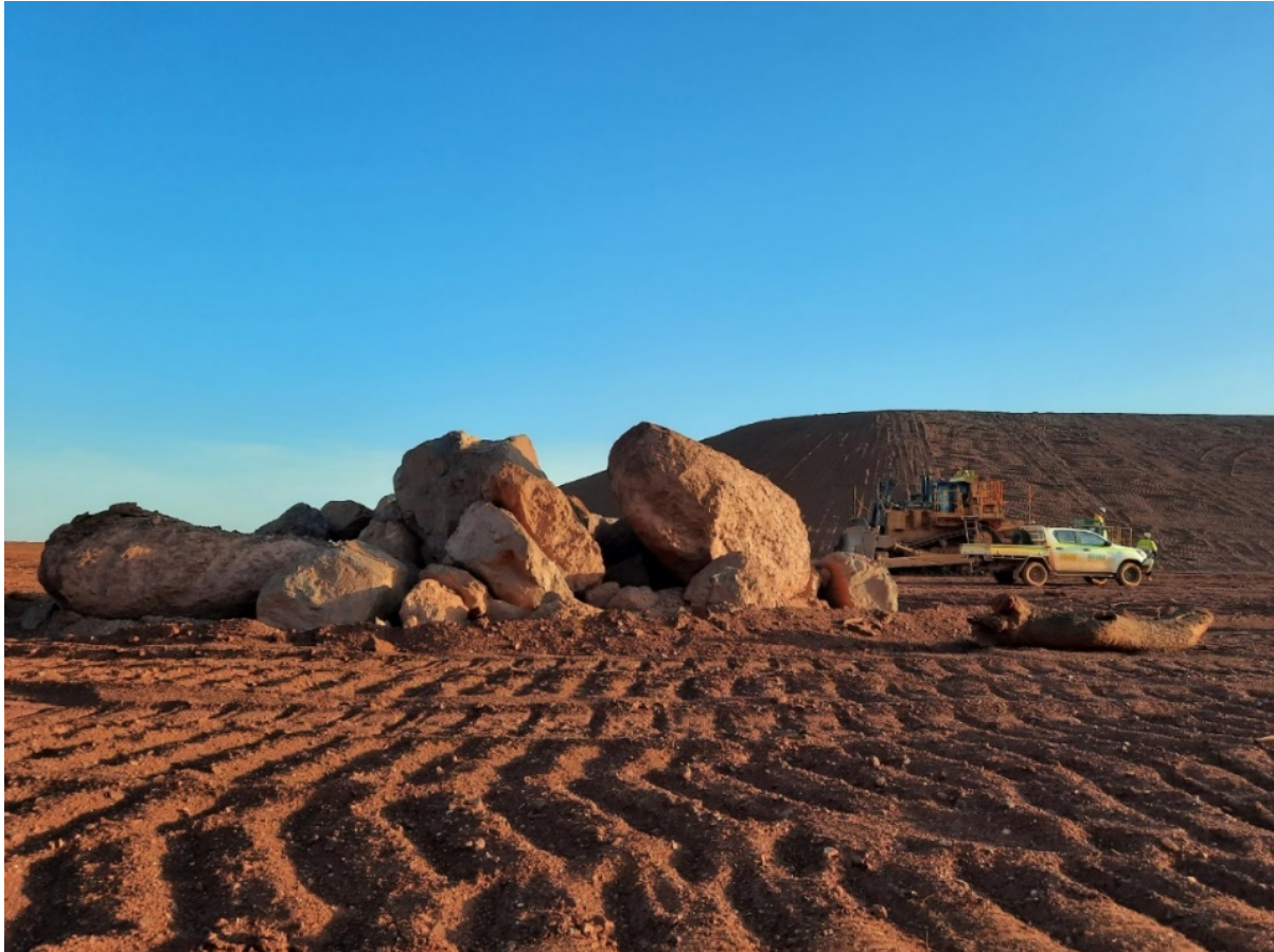
Figure 6 Oversize boulders were placed into rock habitat formations
