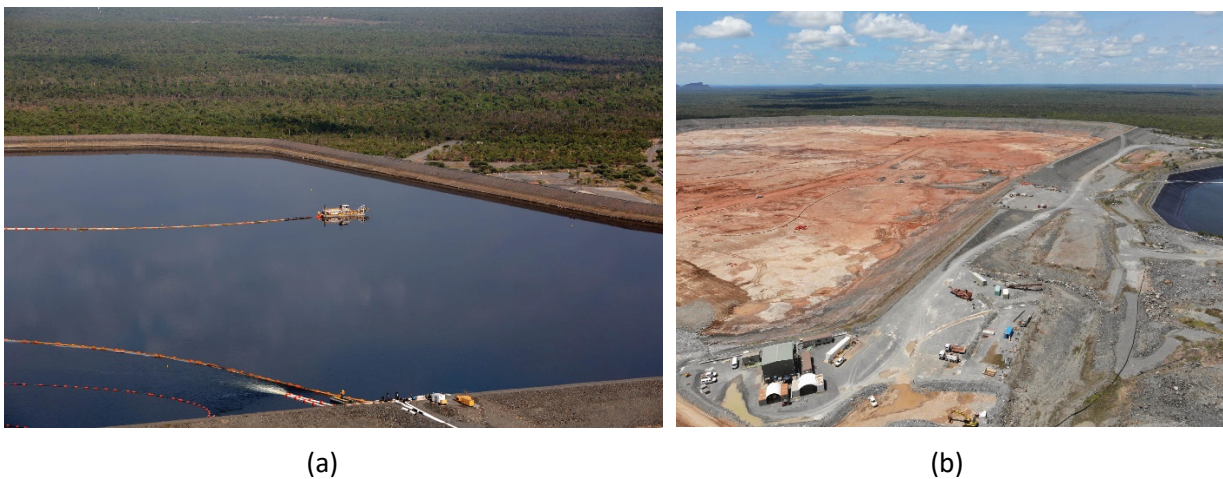
Figure 4 Ranger tailings dam at the commencement of dredging (a) and following all tailings removal (b)
