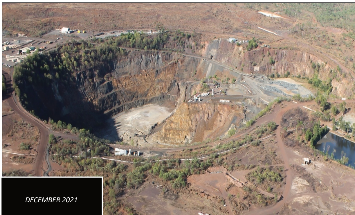
Figure 8 Cosmo Pit pre-backfill
