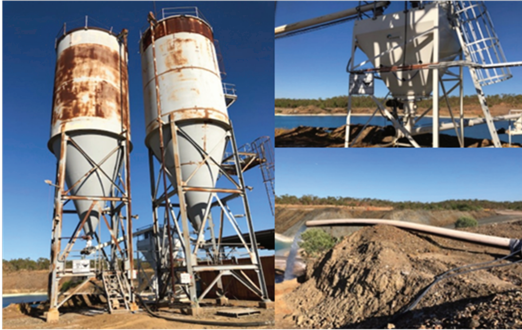
Figure 6 Quicklime inline dosing setup
