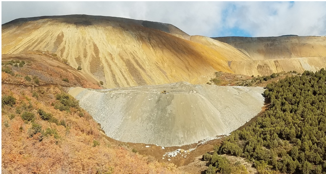
Figure 4 Regrading the lower slopes of the South Dumps
