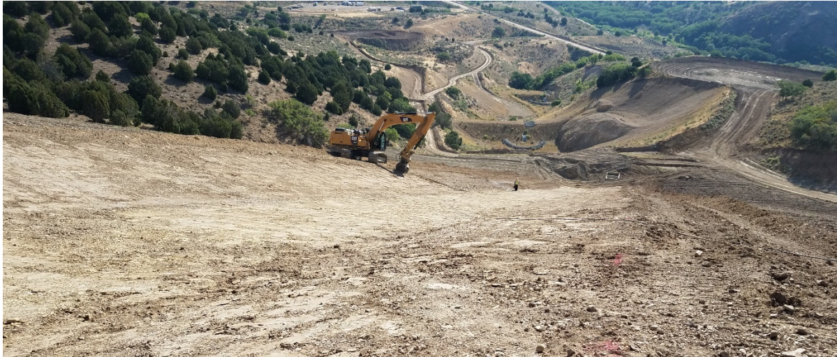
Figure 7 Subsurface grading and compaction preparation of stormwater downdrains
