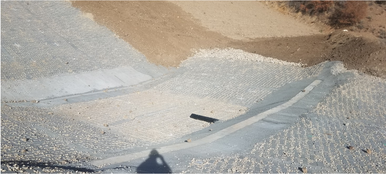
Figure 6 Articulated concrete blocks downdrain, energy dissipator on bench, and catch bench
