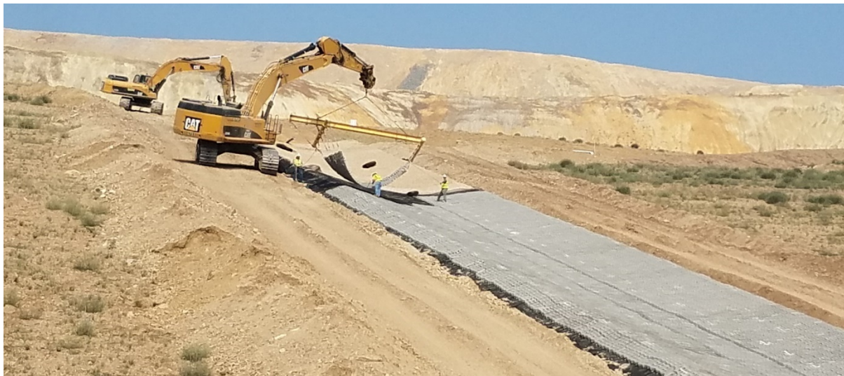
Figure 8 Installation of the articulated concrete block (ACB) revetment in the stormwater downdrains
