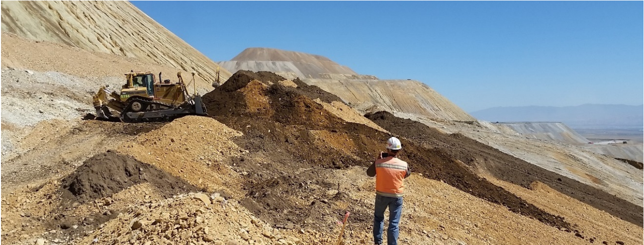
Figure 10 Cover materials are staged in layers by end dumping cover materials in equal parts at the crest of the slope. Material is blended through the dozing process
