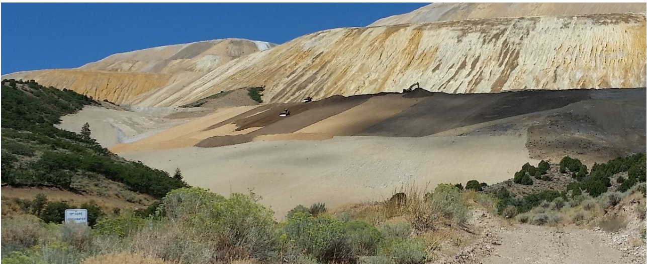
Figure 9 Cover materials are staged in layers by end dumping cover materials in equal parts at the crest of the slope. Material is blended through the dozing process
