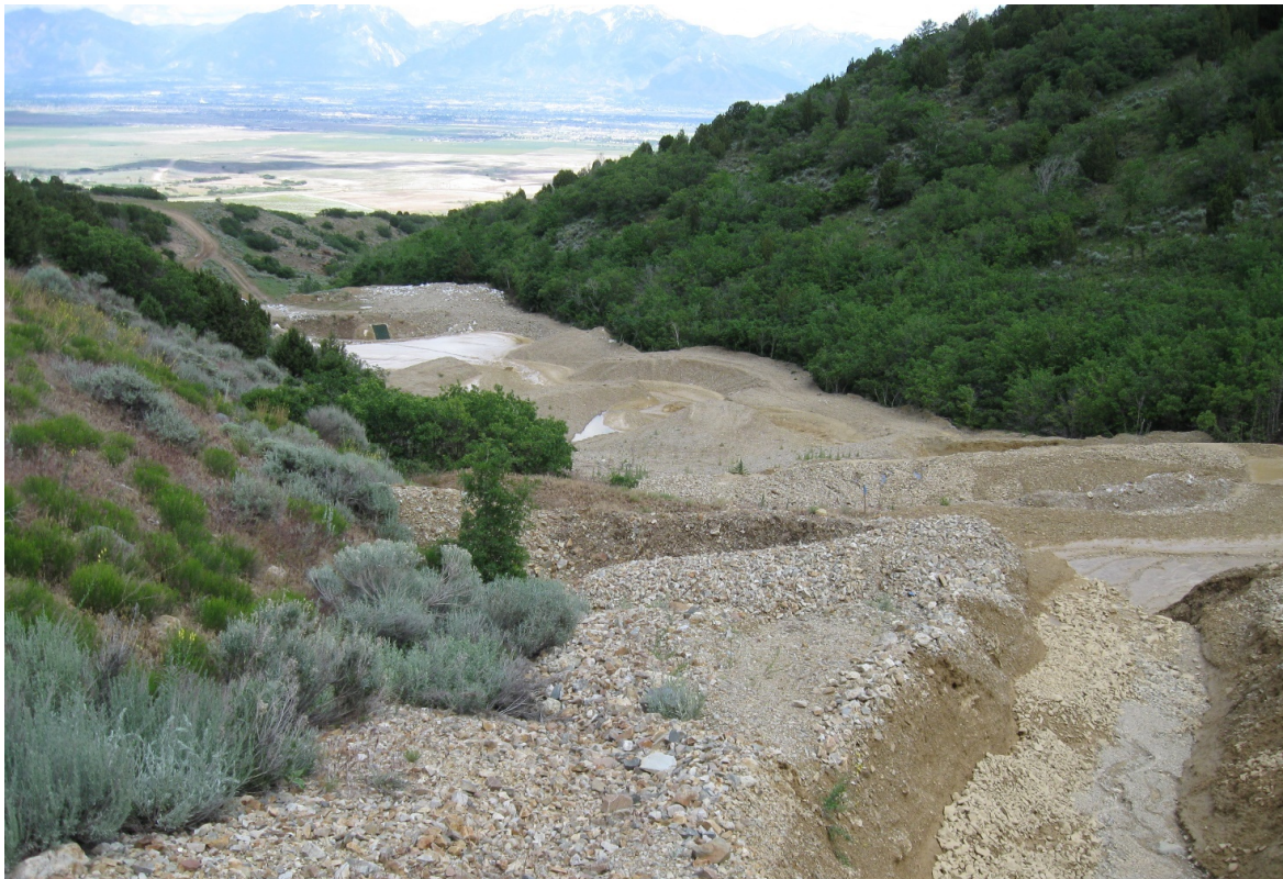
Figure 5 The South Dumps Yosemite drainage detention basin buried after an intense rain event in 2009
