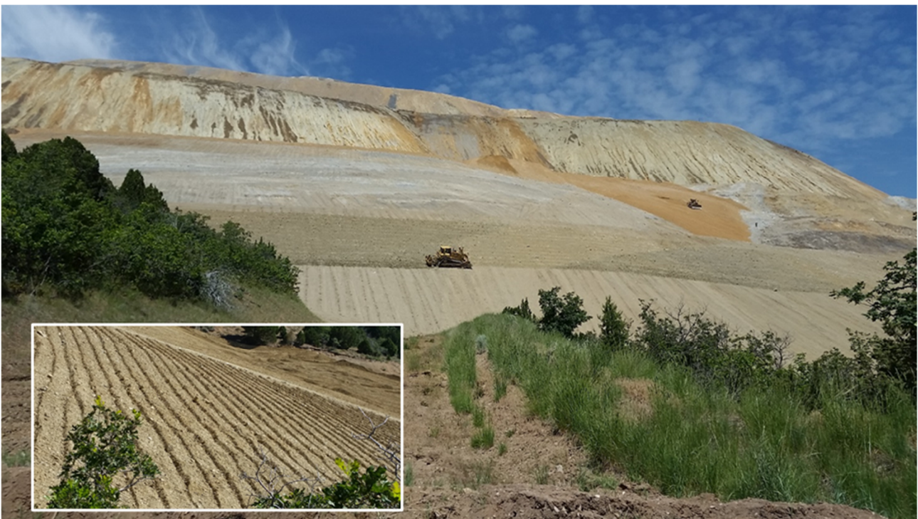
Figure 11 Graded and cross-ripped waste rock in preparation for cover placement
