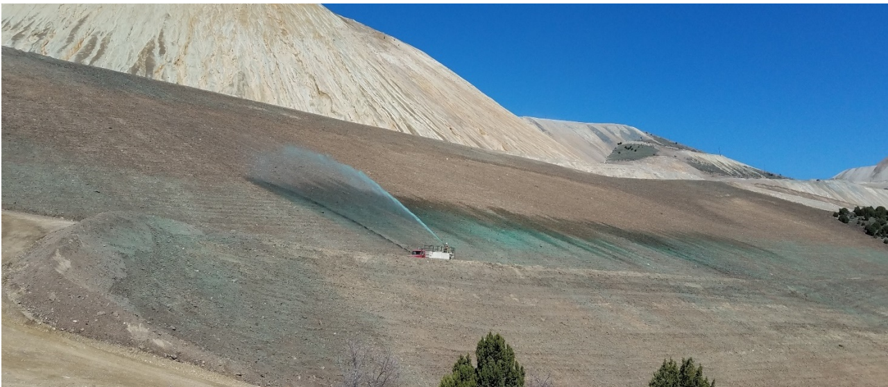
Figure 12 The hydroseed truck moving along the bench and toe of the slope
