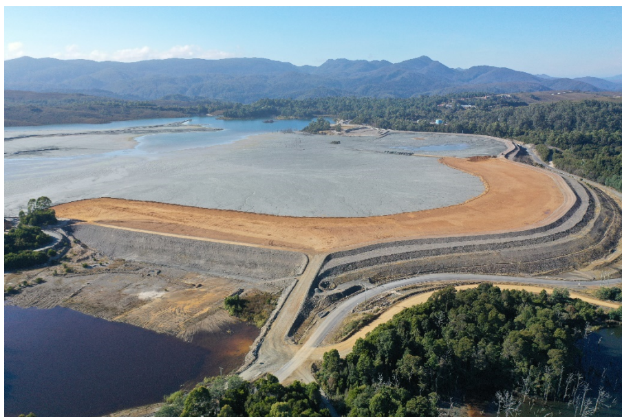
Figure 7 Clay cover placement
