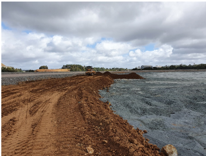
Figure 6 Clay cover placement
