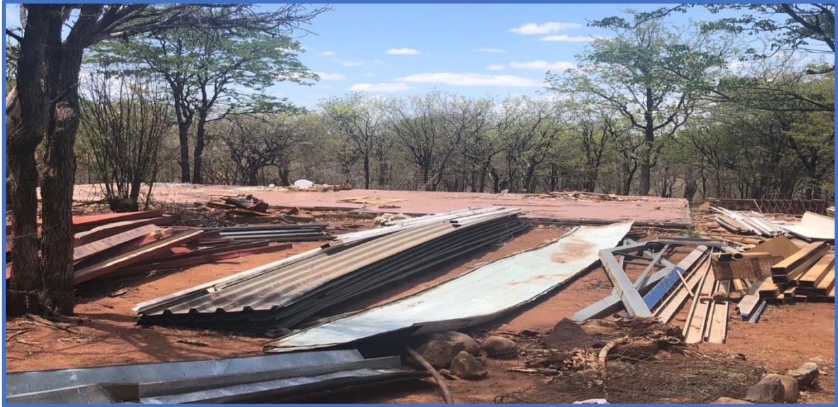
Figure 8 Demolished prefabricated house at Tshikondeni Mine Village
