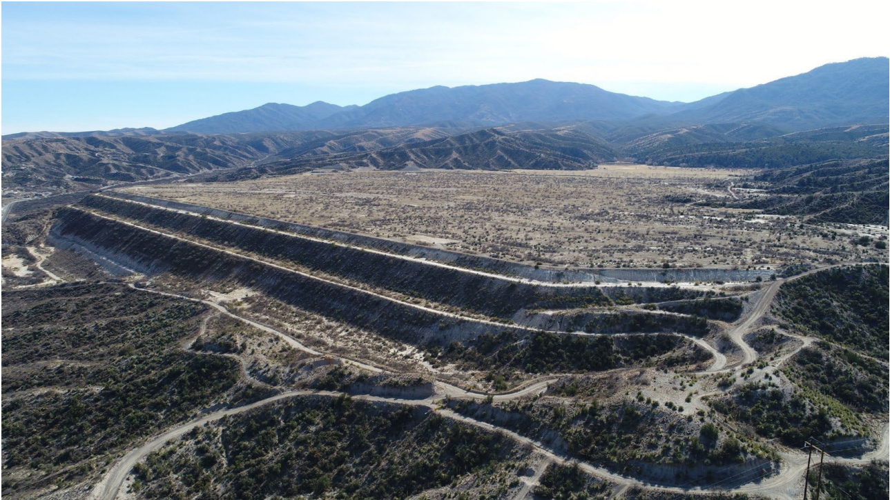
Figure 1 BHP Copper Inc.'s Solitude Tailings Facility was constructed using a starter berm and upstream raises, was operated from 1928-1959, and contains ~116 million tonnes of copper porphyry tailings
