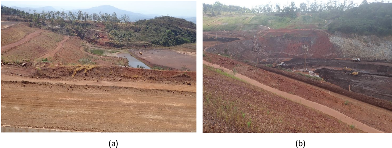
Figure 7 Photographs of B3/B4. (a) PDE X and pond, September 23, 2019; (b) Sump located near original ground level, PDE X, and depth of tailings removal on the left flank, April 18, 2023.
