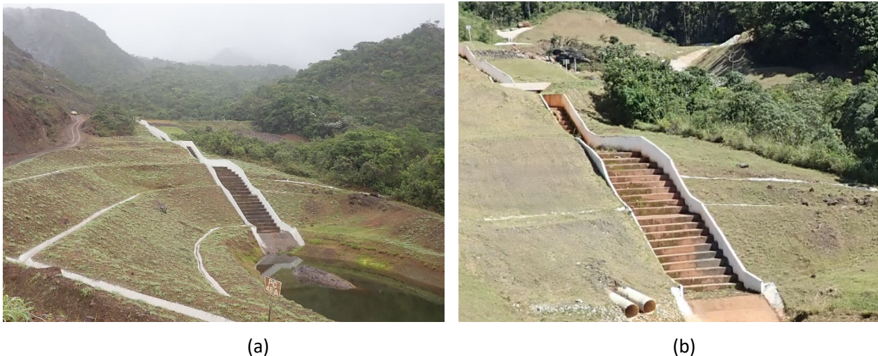
Figure 2 Photographs of Paracatu Dam. (a) Original condition, December 3, 2019; (b) After dam removal May 2, 2023. Note the two buried pipes near the stepped spillway chute.
